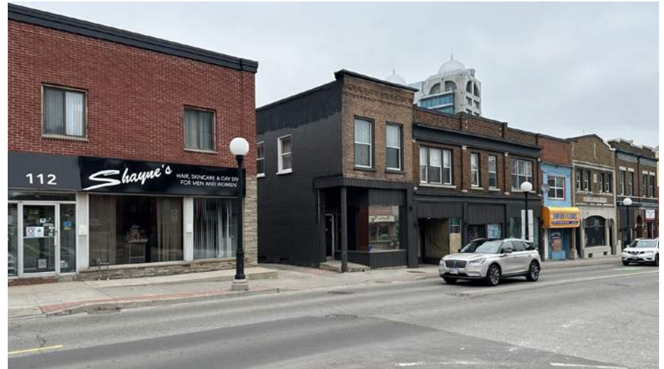
Figure 16. View of neighboring buildings along Queen Street.
