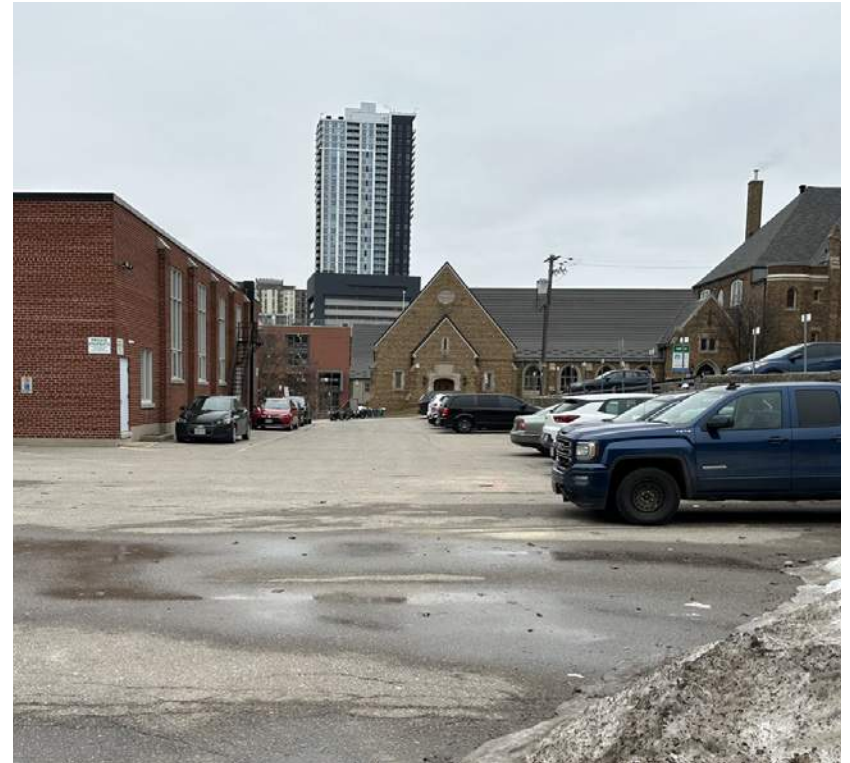
Figure 7. View of the asphalt parking lot at the rear of the site looking north towards Church Street entry/exit to the site.
