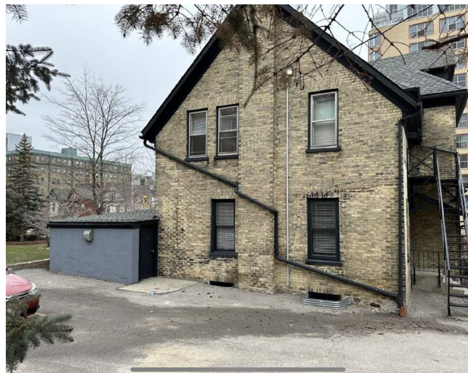
Figure 6. View of the rear heritage property at 149 Queen Street South (left) adjacent to it. The new 6-storey affordable housing building is proposed to be constructed behind this rear facade.
