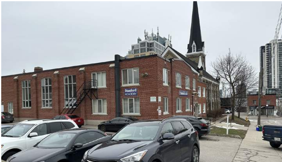
Figure 12. View of rear of the property looking northwest from Church Street.
