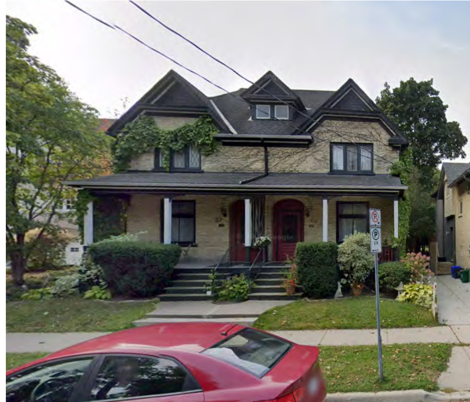
Not sure if this image could be helpful for us somewhere '67 – 69 Ahrens – two semis cooperating' from pg 22 of the Heritage report
