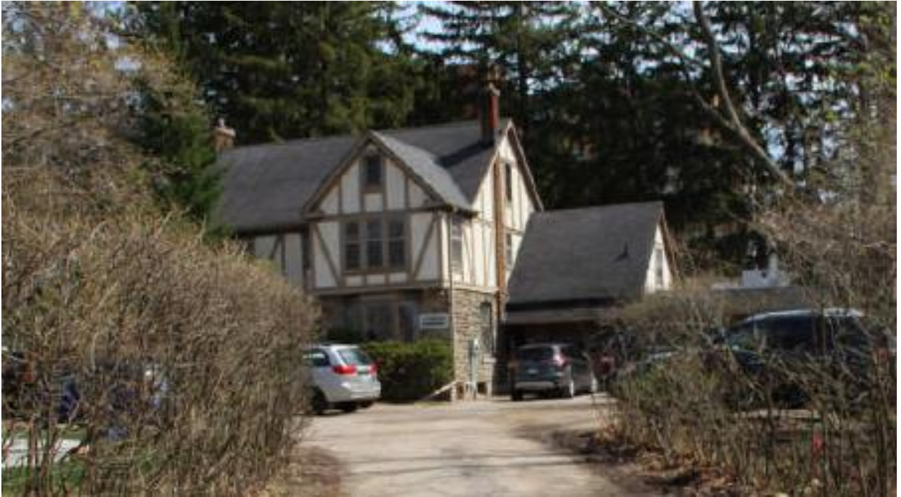
Figure 3: Front elevation of 35 Sheldon Avenue North
