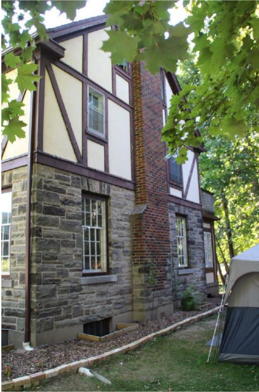
Figure 8: West Elevation of 43 Sheldon Avenue North
