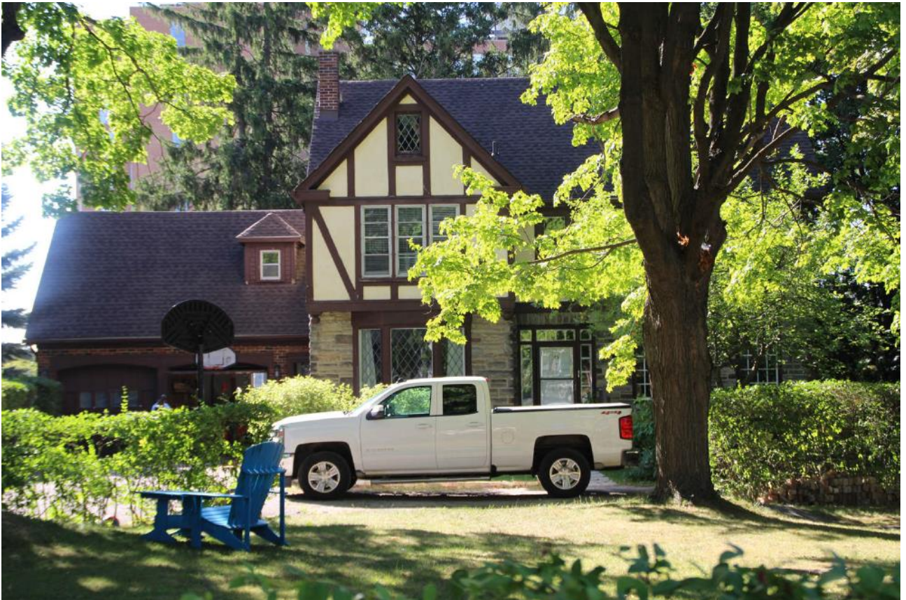
Figure 7: Front elevation of 43 Sheldon Avenue North
