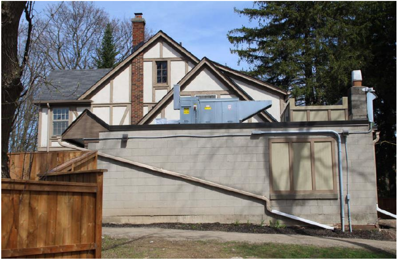
Figure 4: West elevation of 35 Sheldon Avenue North
