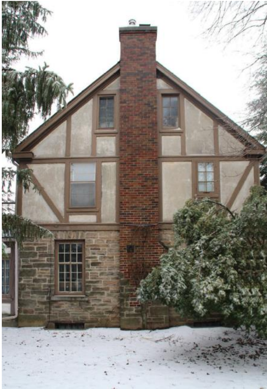
Figure 5: East elevation of 35 Sheldon Avenue North
