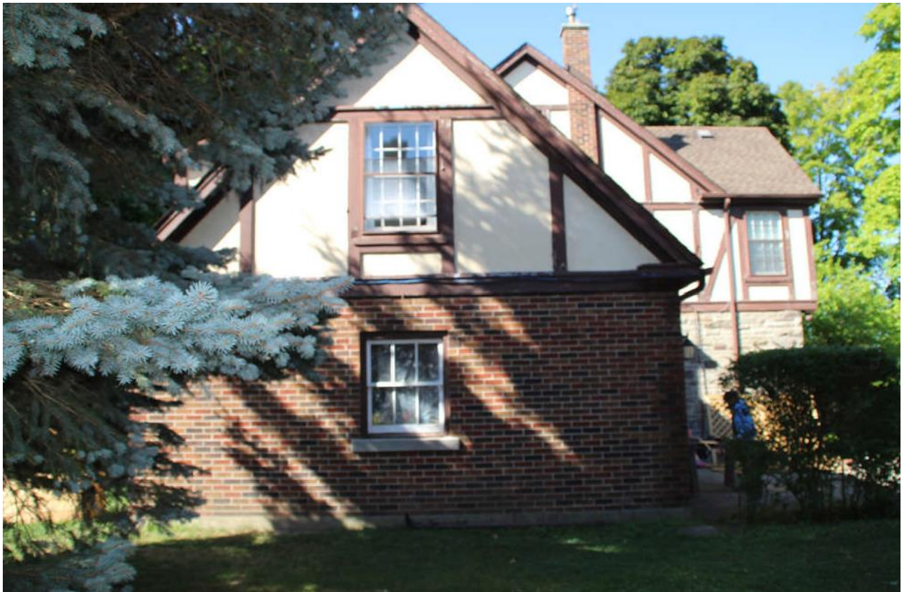
Figure 10: East elevation of 43 Sheldon Avenue North
