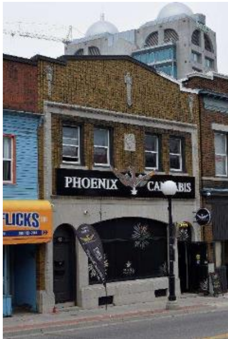
Figure 2. Front Façade of 90-92 Queen Street South.
