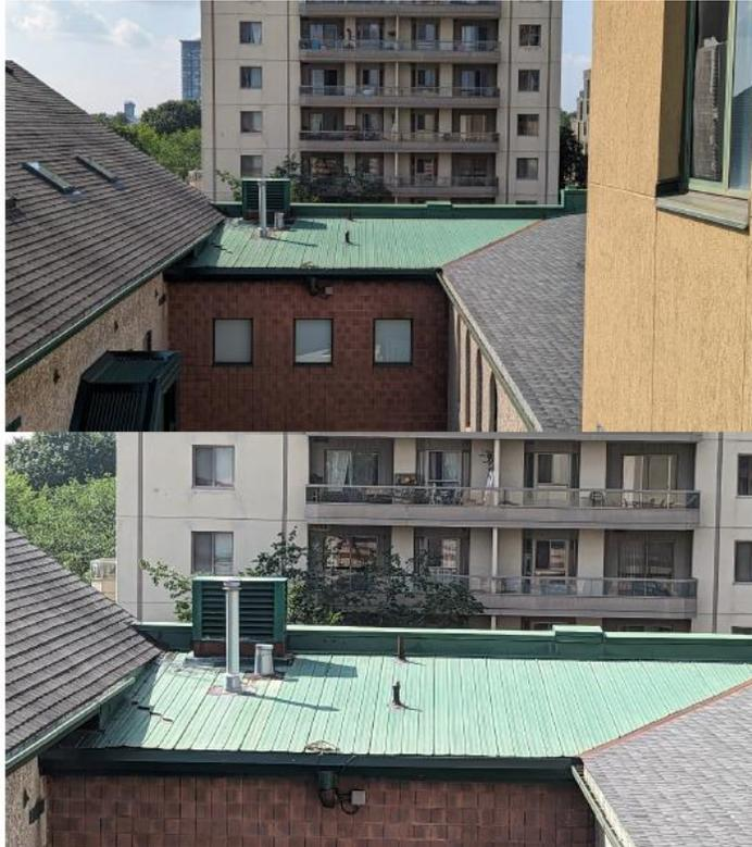
**Figure 4: Existing corrugated metal roof (images provided by owner/applicant)**
