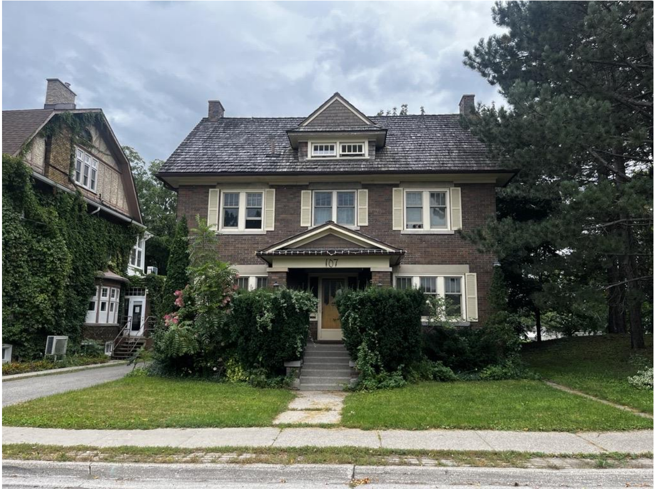
Figure 2: Front Facade of Subject Property
