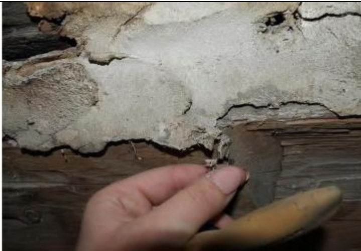
Detailing of chinking between logs (mortar with horsehair) (source: MHBC Planning, 2018)
