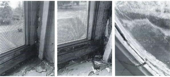
Figure 4: Images of Existing Windows Showing Deterioration
