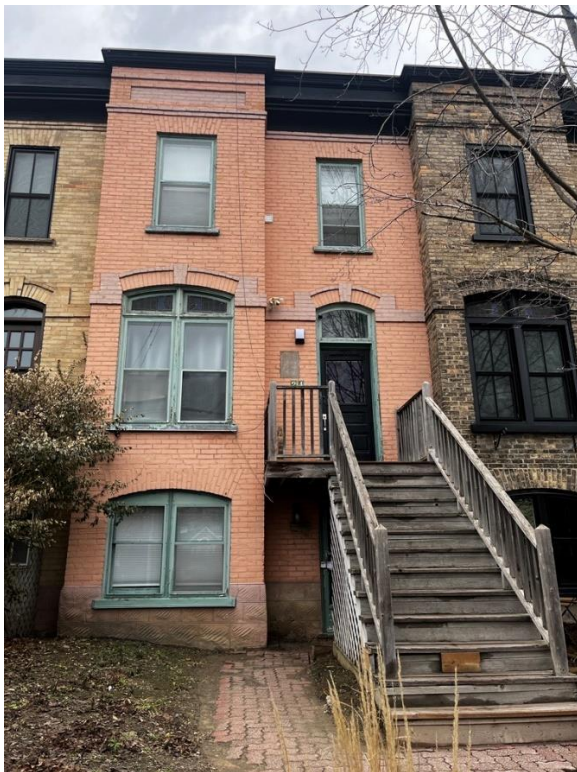
Figure 2: Front Façade of 24 Courtland Avenue East
