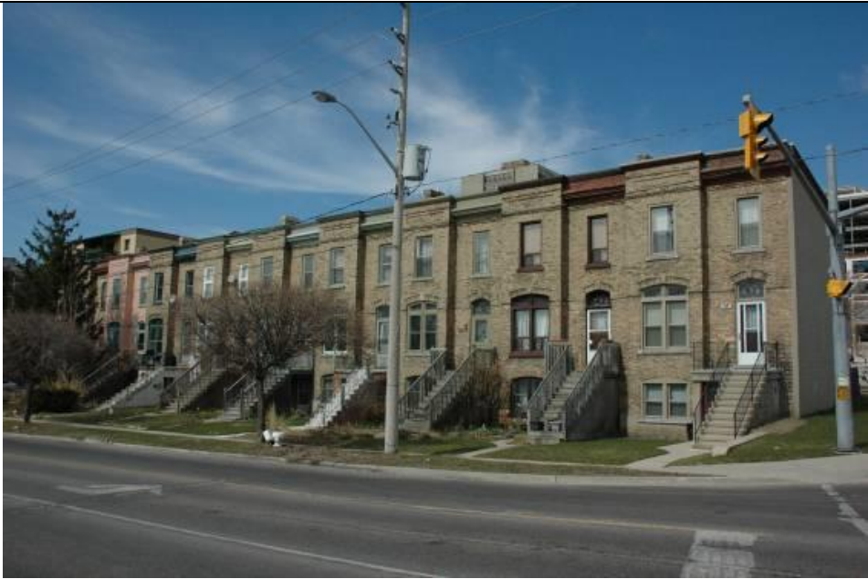
24 Courtland Avenue East – Entire Nelson Terrace Row House Building
