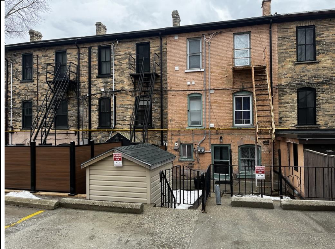
Rear Façade of 24 Courtland Avenue East
