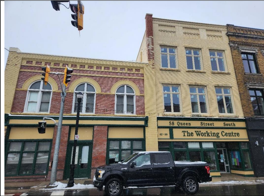
58 Queen Street South – Front (East) Façade
