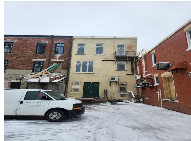
58 Queen Street South – West (Rear) Façade
