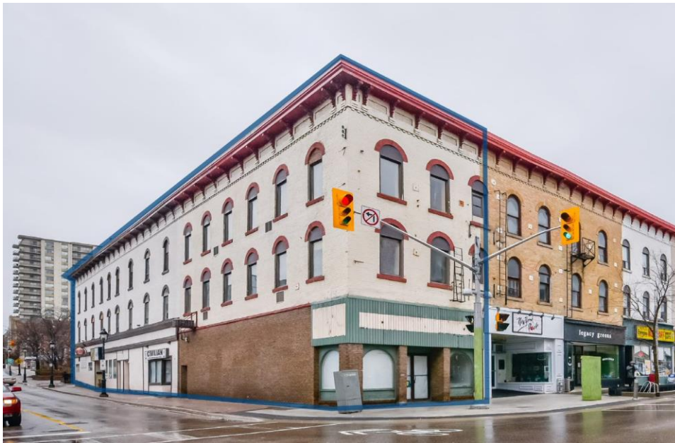
Figure 3: 4 King Street East/1 Queen Street North Before Restoration
