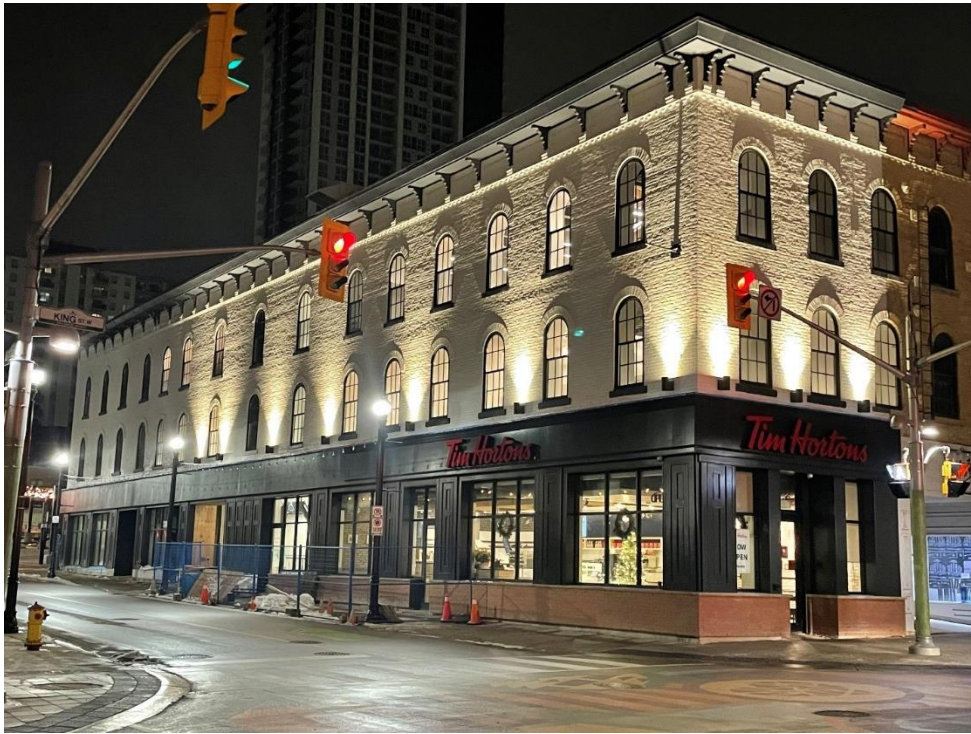
Figure 2: 4 King Street East/1 Queen Street North After Restoration
