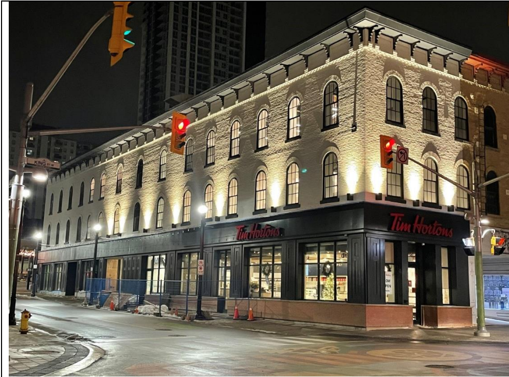
4 King Street East/1 Queen Street North – Front (South) and Side (West) Façade
