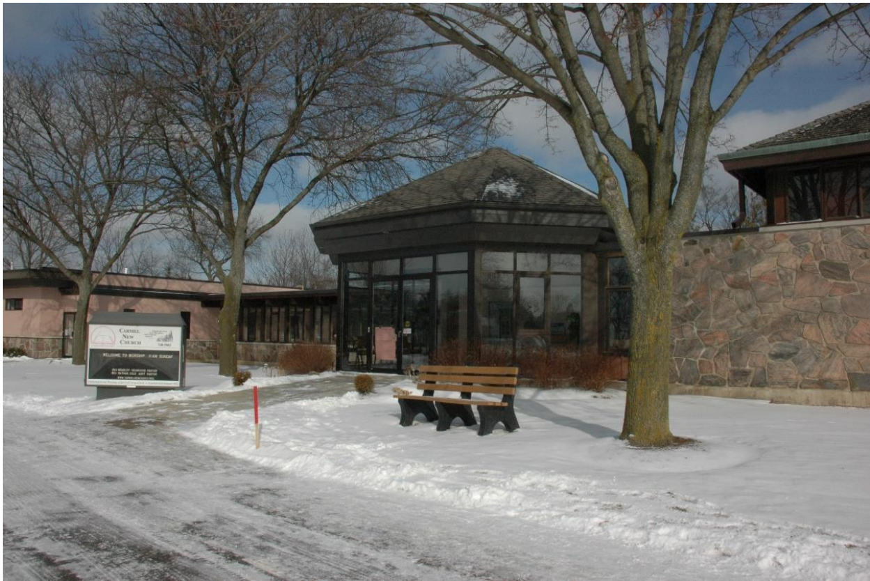
Figure 4: Western Portion of the Building Encompassing the New Addition and School
