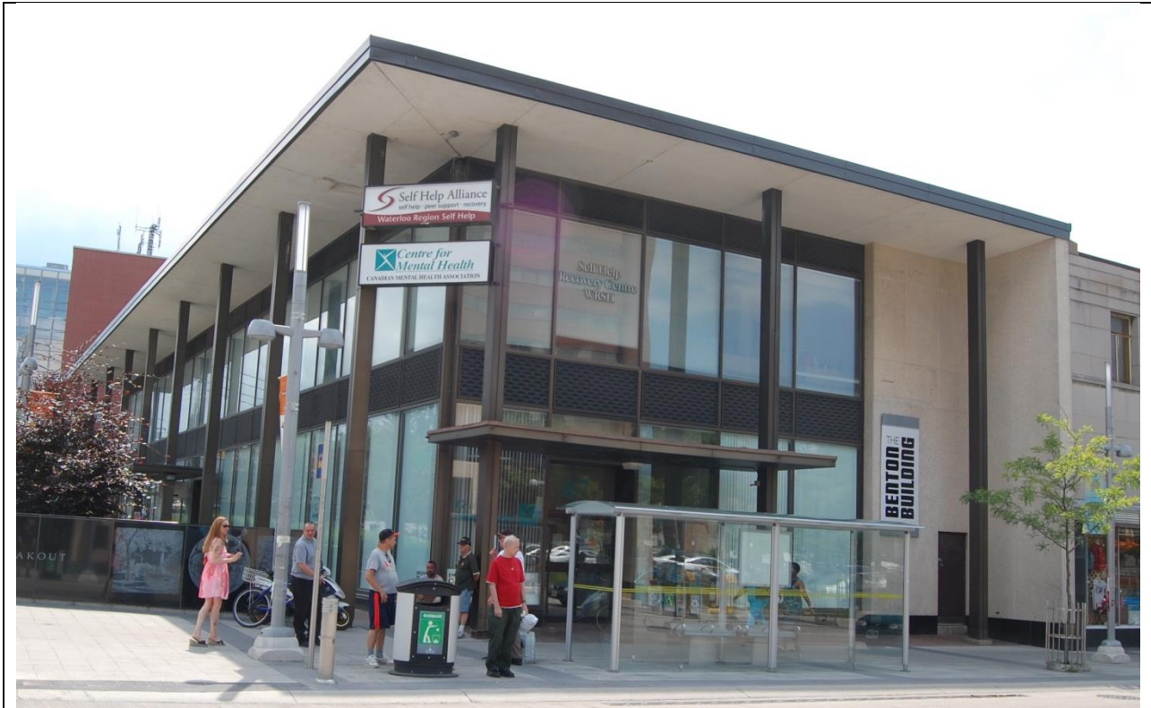
67 King Street East – Front Elevation
