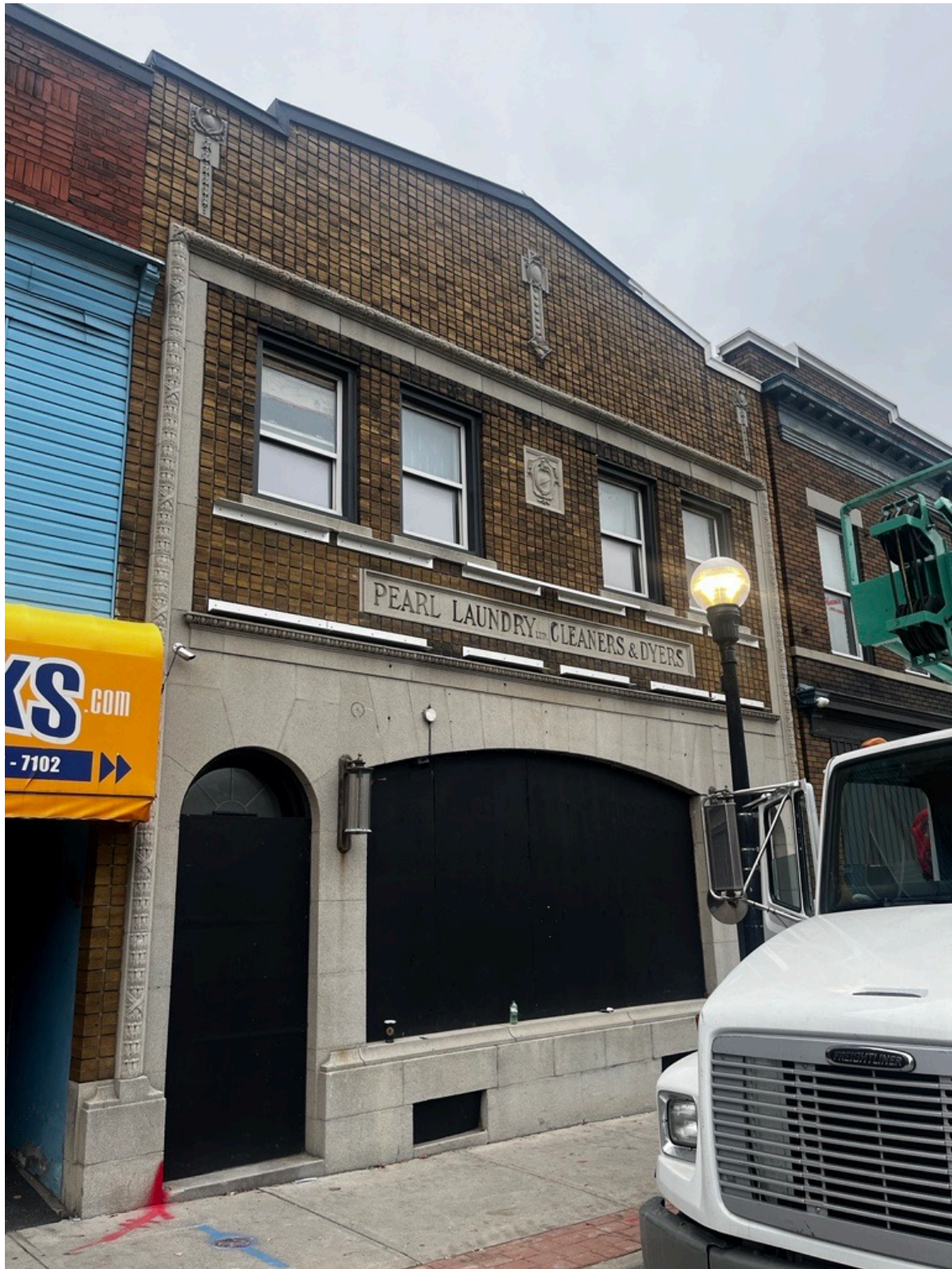
Figure 2: Front façade of 90-92 Queen Street South
