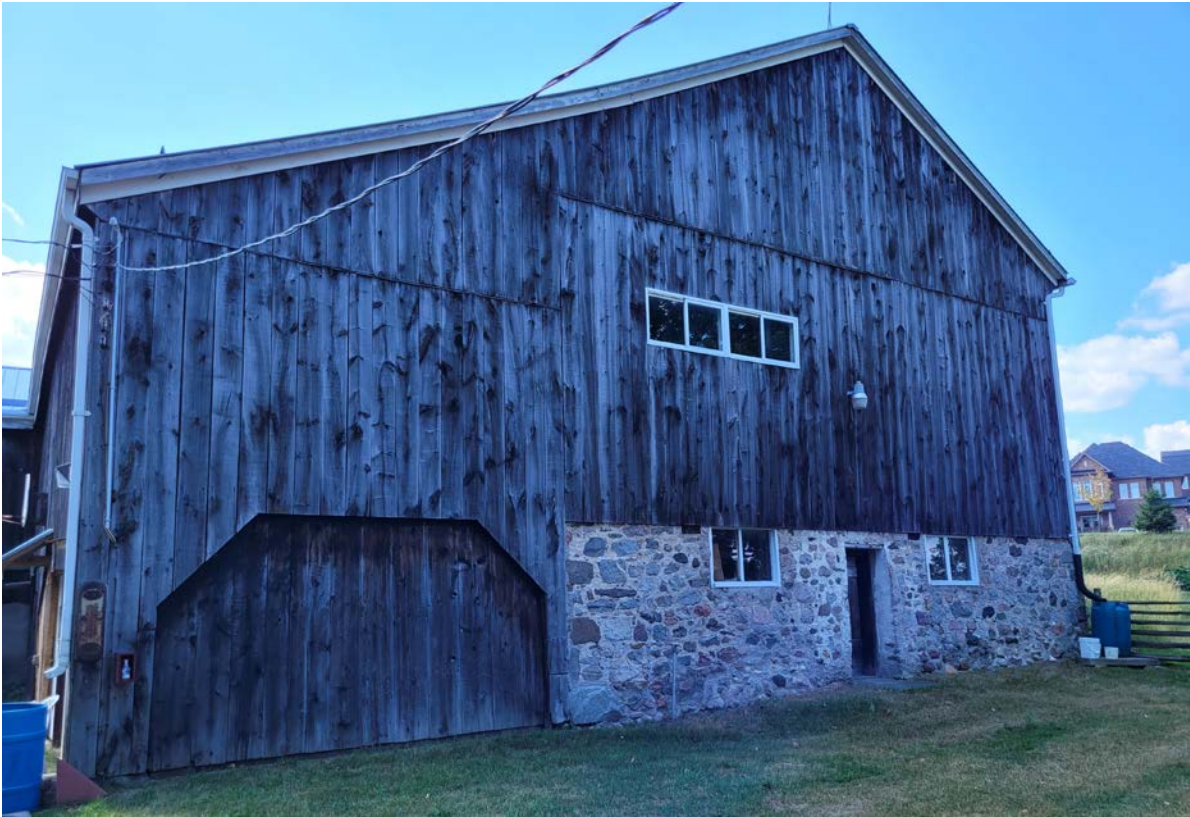
Figure 5: View of Barn (photo provided by MHBC)
