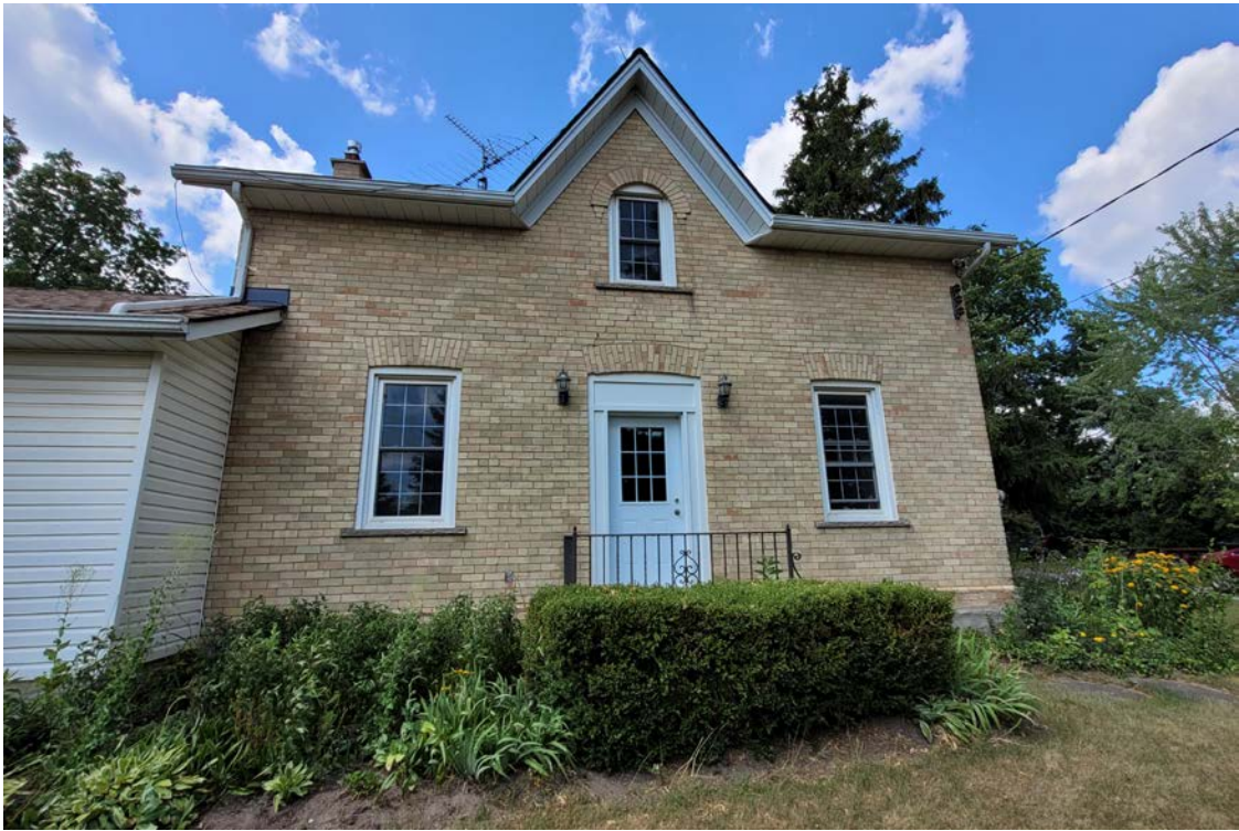
Figure 2: South (Front) Façade of Farmhouse (photo provided by MHBC)
