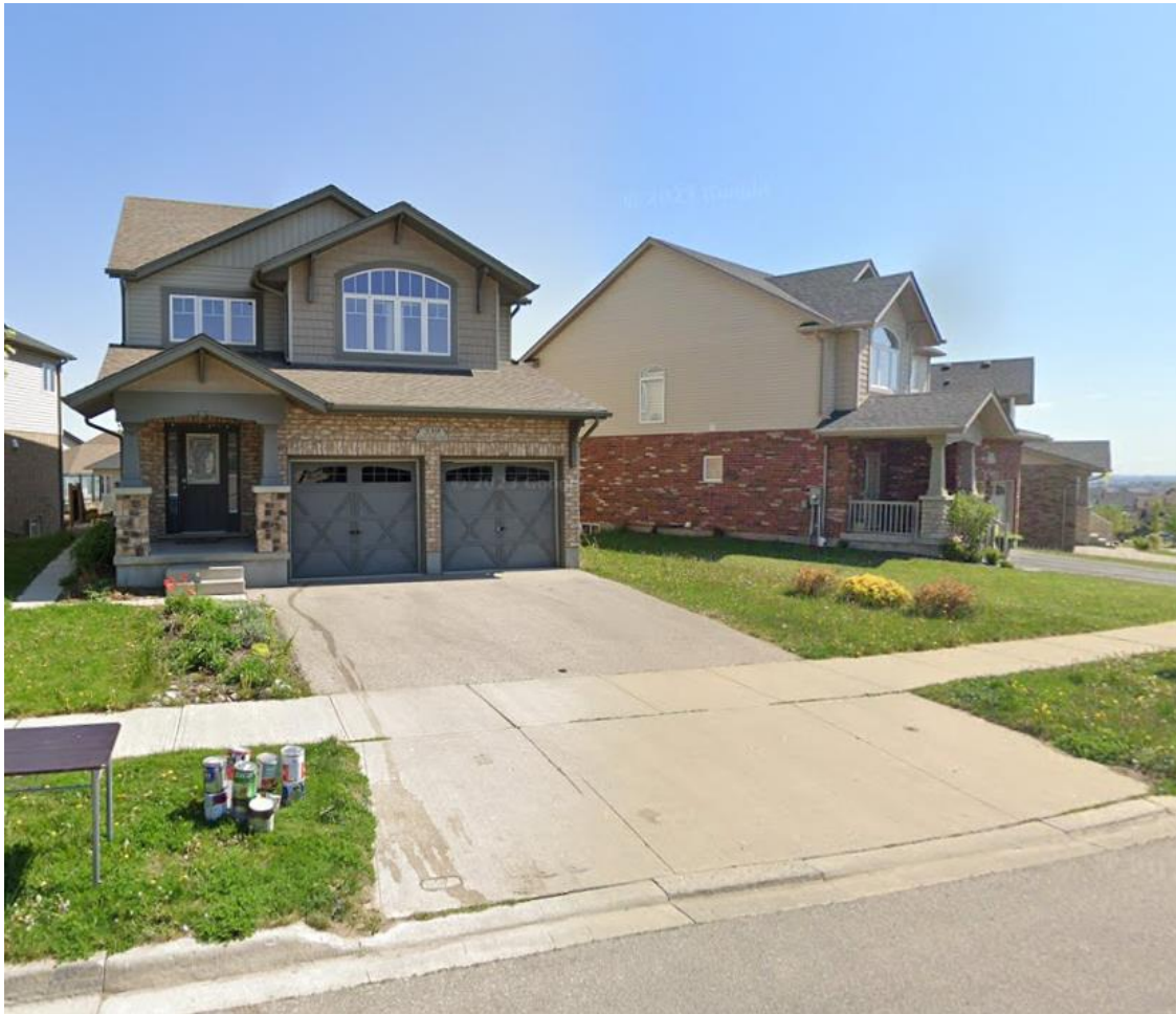
Figure 7 – Detached home on Gravel Ridge Trail
