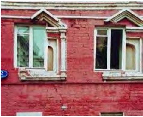
Figures 40 & 41: (left) View of altered window opening at the east elevation of Section "A" of the building, (right) Sample of inappropriate window and window opening alterations.
