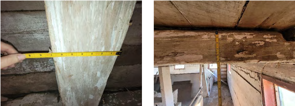
Figures 62 & 63: Dimensions of typical timbers within the barn, (Source: MHBC, 2023)
