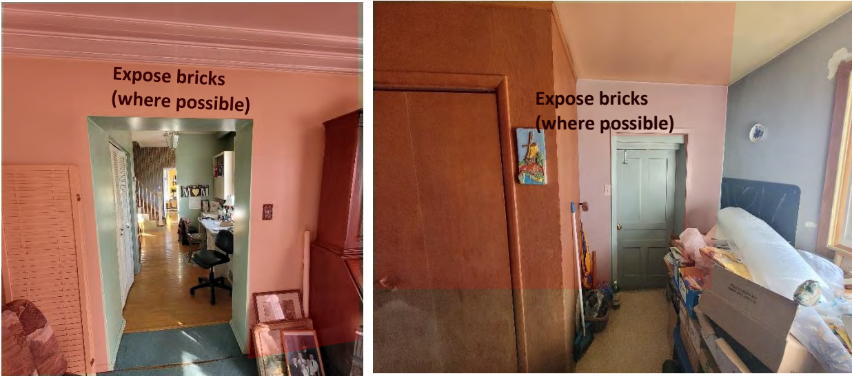
Figures 32 & 33: (left) View door opening "B" (west elevation) noting approximate area where brick may be exposed after contemporary materials are removed, (right) View of door opening "A", looking south, noting area where brick may be exposed (shaded in red) (Source: MHBC, 2023)
