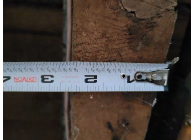
Figures 12 & 13: (left) Detail view of internal sawn beam, approximately 9" wide, (right) Detail view of interior basement floor joist, approximately 2 1/4" wide, (Source: MHBC, 2022)
