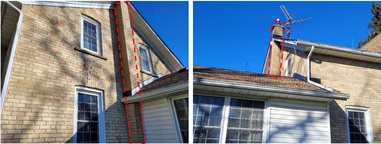
Figures 29 & 30: (left) View of west elevation of Section “A” noting 20 th century chimney proposed for removal, (right) View of north elevation of Section “B” noting 20 th century chimney proposed for removal, (Source: MHBC, 2023)
