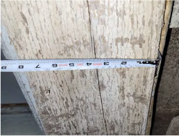
Figures 12 & 13: (left) Detail view of internal sawn beam, approximately 9" wide, (right) Detail view of interior basement floor joist, approximately 2 1/4" wide, (Source: MHBC, 2022)
