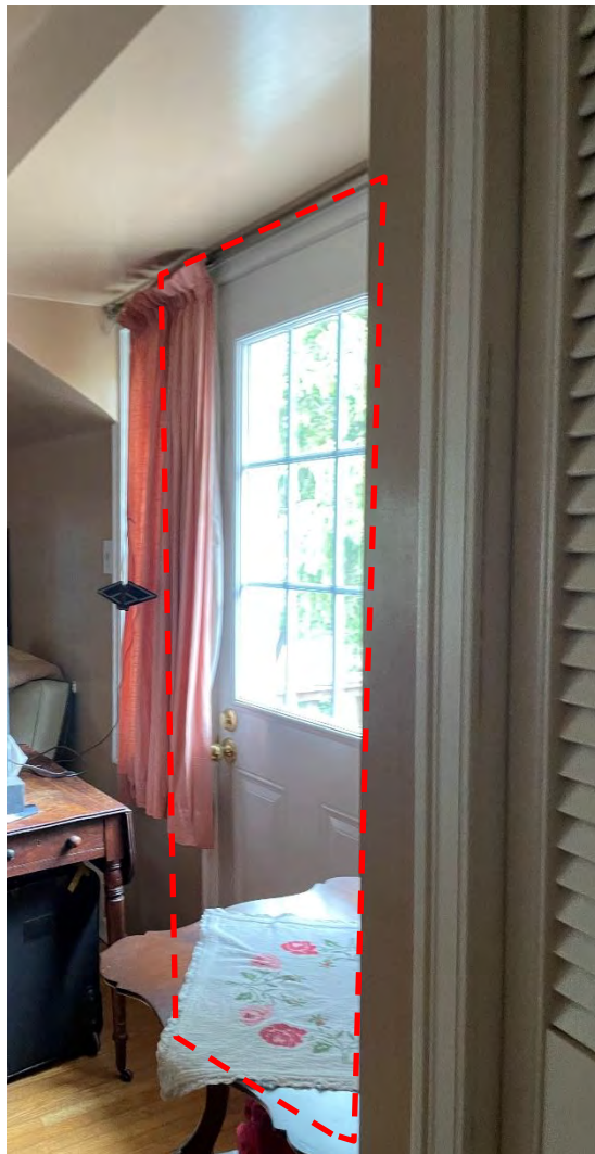
Figures 28: View of door opening to be exposed following the removal of Section "F", at the east elevation of Section "B" (Source: MHBC, 2023)
