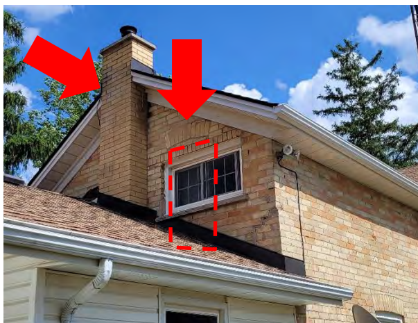
Figures 9 & 10: (left) View of north elevation (note exterior chimney and altered window opening). Approximate location of original window opening outlined with red dashed line. (right) Detail view of east elevation (ground floor), (Source: MHBC, 2022; MHBC, 2023)
