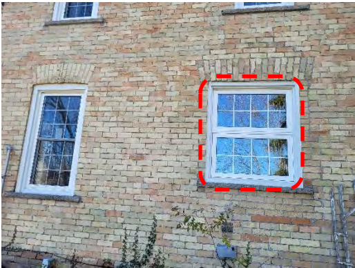
Figures 40 & 41: (left) View of altered window opening at the east elevation of Section "A" of the building, (right) Sample of inappropriate window and window opening alterations.
