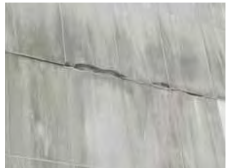
Masonry used on the exterior of modern buildings is generally a cladding attached to a separate structure. Clips, anchors or shelf angles are used to attach the stone panels or brick masonry. The deterioration of these anchors is an area of potential deterioration and failure. Monitoring the condition of these anchors is a vital part of a maintenance plan, as their failure can lead to very significant damage.
