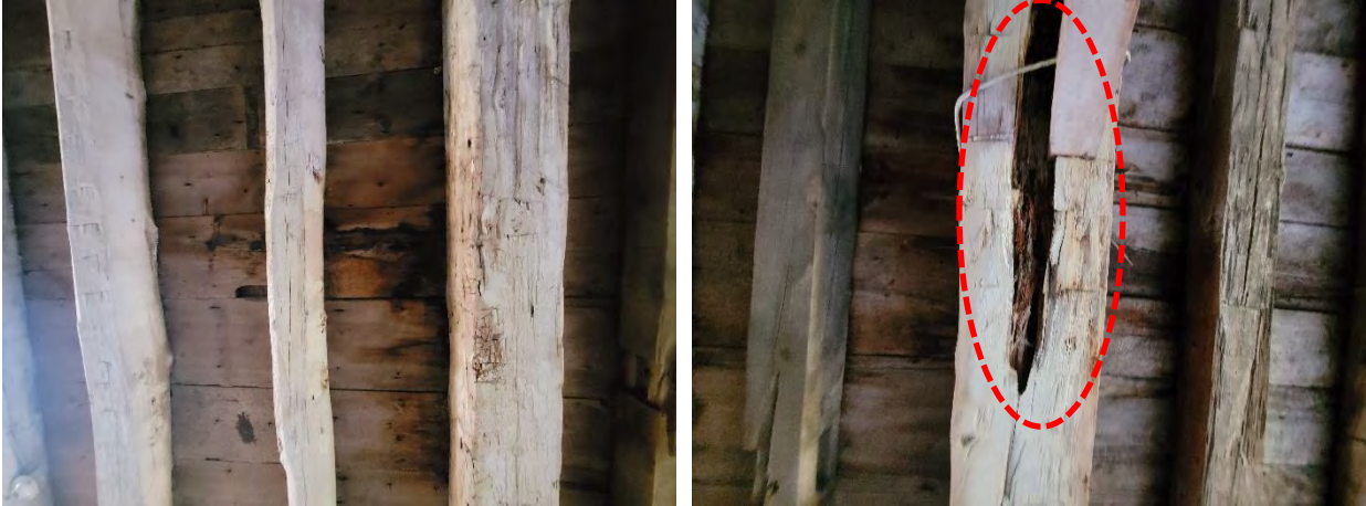
Figures 60 & 61: Photographs of typical timbers within the barn, (Source: MHBC, 2023)
