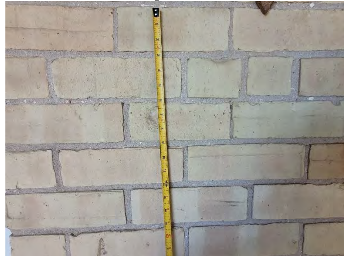
Figures 7 & 8: (left) Detail view of brick dimensions, colour and patina at original portion of the dwelling (noting colour differences (yellow, terra cotta coloured bricks)) (right) Detail view of brick dimensions, colour and patina at rear summer addition (noting colour differences from original portion of the dwelling) (Source: MHBC 2023)
