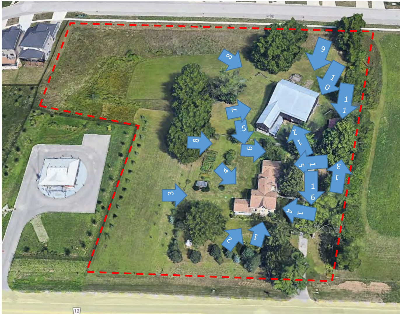
Figure 1: Aerial photograph of subject property at 628 New Dundee Road noting approximate location of photos taken. (Source: GoogleEarthPro, accessed 2022)
