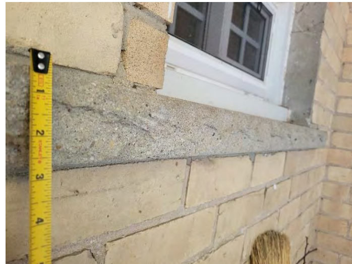
Figures 3 & 4: (left) View of contemporary window opening and contemporary window at south elevation of original portion of the dwelling, (right) Detail view of rusticated concrete sill at south elevation of original portion of the dwelling (contemporary window opening noted in Figure 3), (Source: MHBC 2023)
