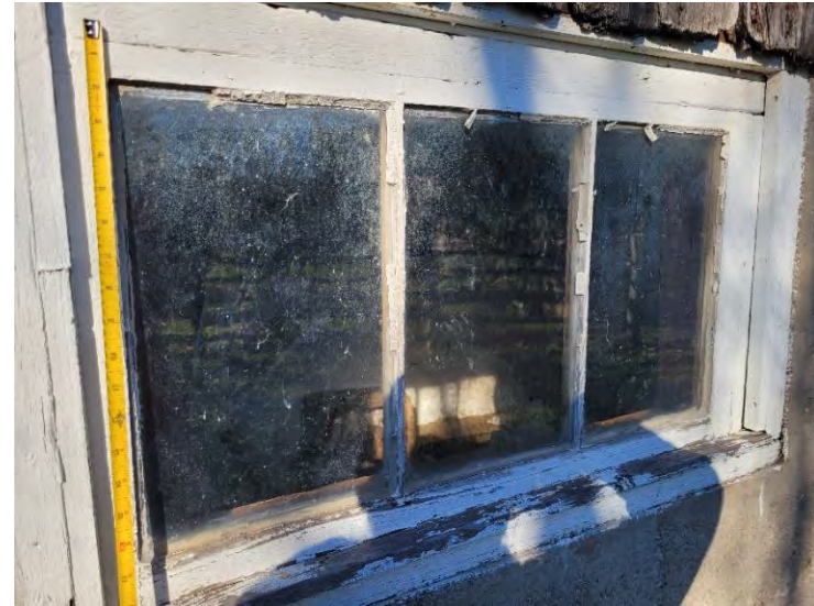
Figures 9 & 10: (left) View of east and partial north elevation, looking south-west, (right) Detail view of 20 th century barn window, noting poor conditions,(Source: MHBC 2023)
