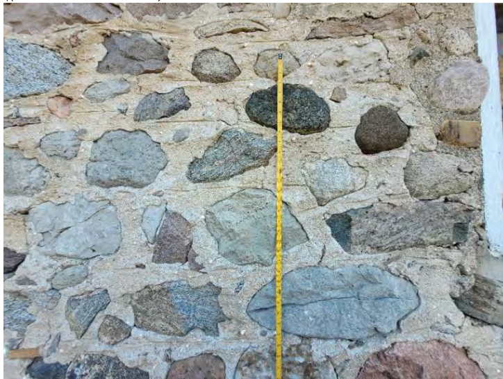
Figures 11 & 12: (left) Detail view of typical barn foundation material and field stones (right) View of concrete foundation at west elevation, (Source: MHBC 2023)
