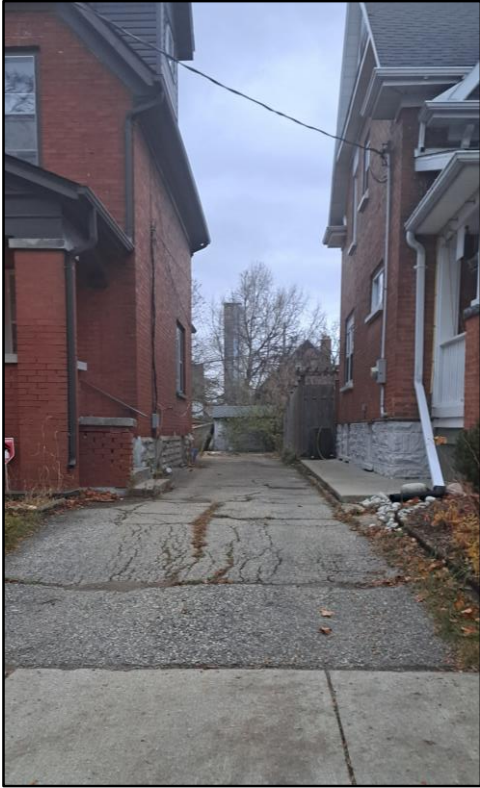
Figure 6 - The Existing driveway on the north side yard
