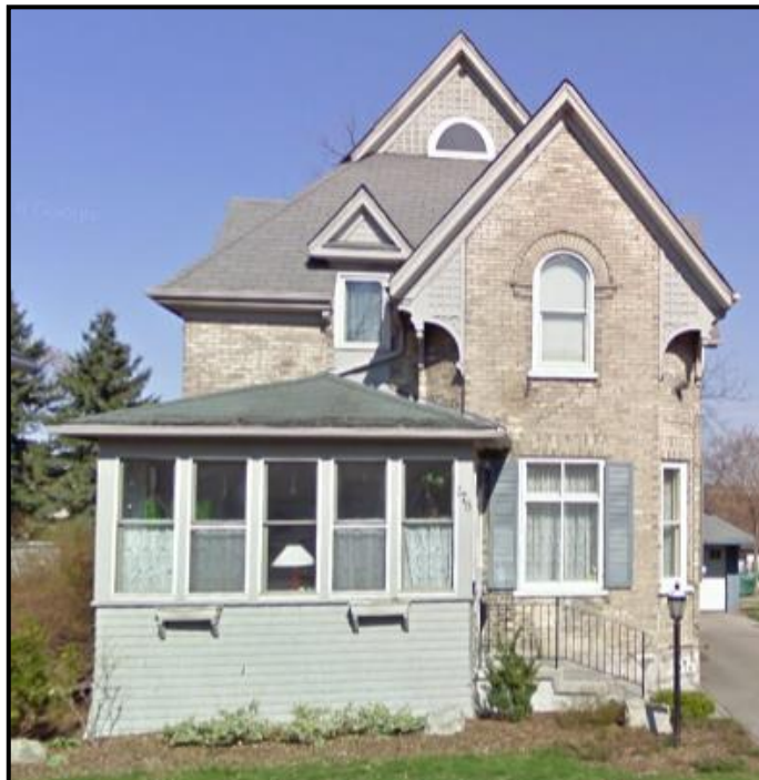
House featured in City's emblem for the Heritage District
