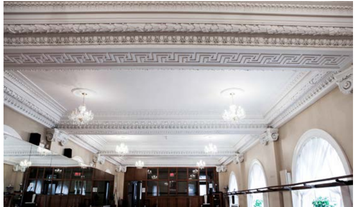
Economical's main office ceiling, c. 1920 and 2012, an enduring catalogue of classical motifs in plaster: Ionic capitals, Greek key, acanthus, imbricated laurel leaves, egg and dart, bead and reel. TOP: photos courtesy of Economical Insurance. BOTTOM: photos by author.
