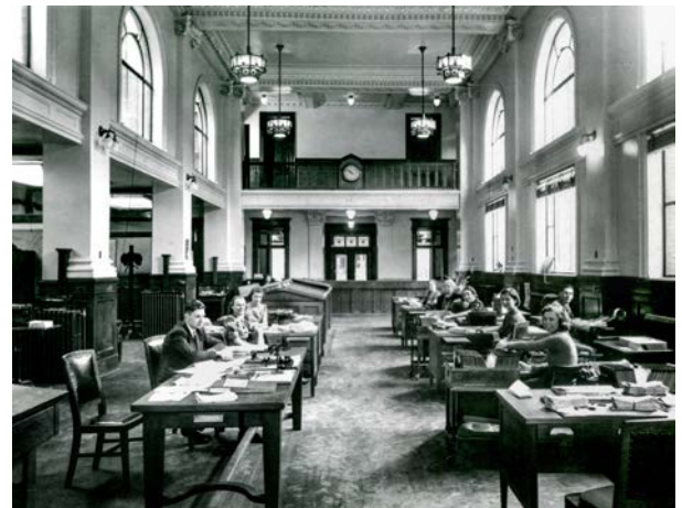
The soaring main office space at Economical in the 1940s, just prior to its division into two floors. In 2021, much survives of the finishes shown here. Courtesy of Economical Insurance.
