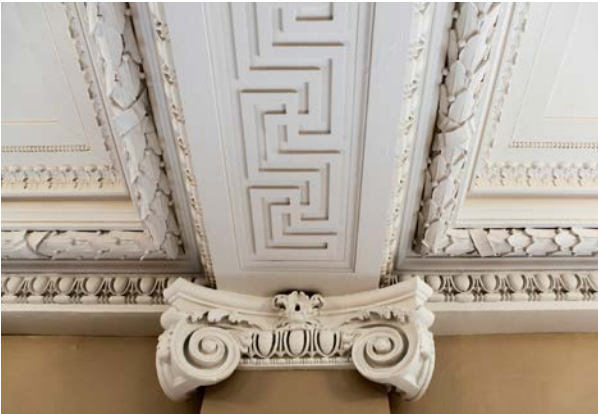
Economical's main office ceiling, c. 1920 and 2012, an enduring catalogue of classical motifs in plaster: Ionic capitals, Greek key, acanthus, imbricated laurel leaves, egg and dart, bead and reel. TOP: photos courtesy of Economical Insurance. BOTTOM: photos by author.
