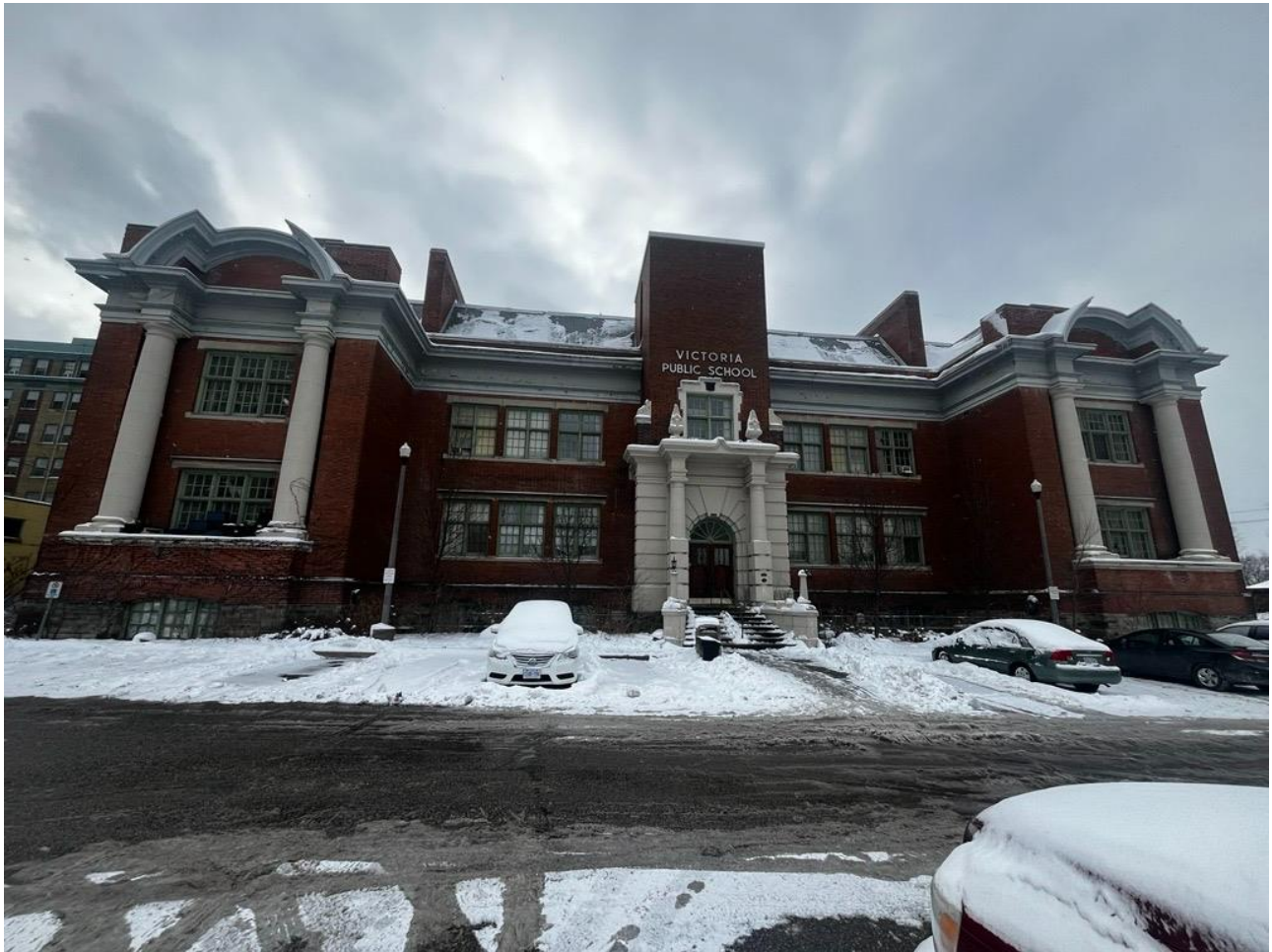
Figure 2: Front Facade of Subject Property
