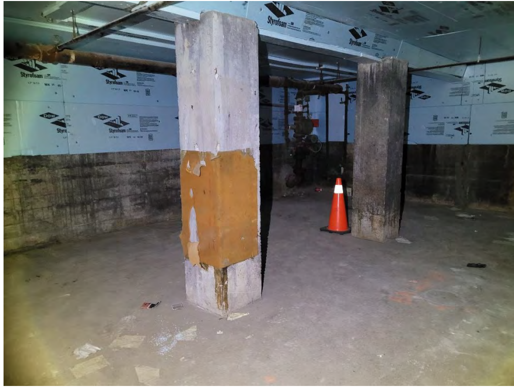
Photo 13: (left) View of utility room, looking south-west, (Source: MHBC, 2023)
