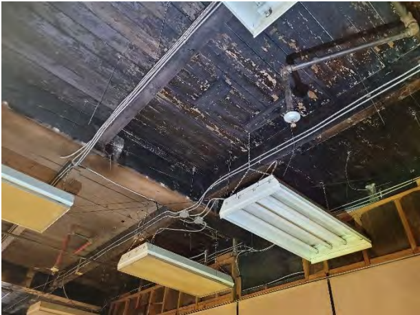
Figures 18 & 19: (left) View of open area, looking south-west, (right) Detail view of ceiling noting fire damage, (Source: MHBC, 2023)
