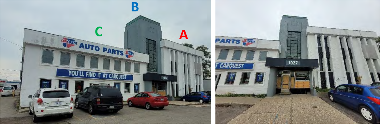
Figures 6 & 7: (left) View of north elevation looking south towards the front elevation of sections "A", "B", and "C", (right) Detail view of the front elevation, looking south towards Section "B", (Source: MHBC, 2023)
