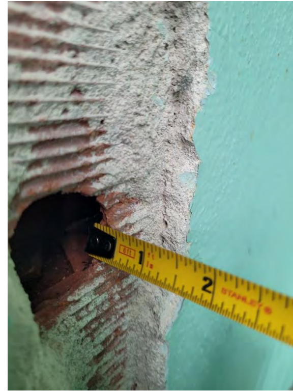
Photos 9 & 10: (left) View of roof access, looking east from access to second level within Section "C", (right) Detail view of hollow terra cotta bricks within Section "B", (Source: MHBC, 2023)
