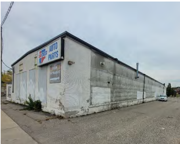
Figures 10 & 11: (left) View of east elevation, looking north-west from Charles Street East, (right) Detail view of east elevation (Section "C") and spray foam and stucco over industrial windows , (Source: MHBC, 2023)
