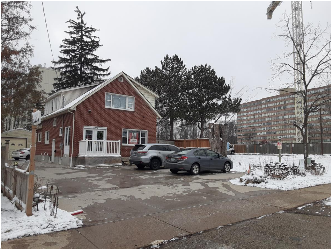
Figure 2 - View from left side of property.
