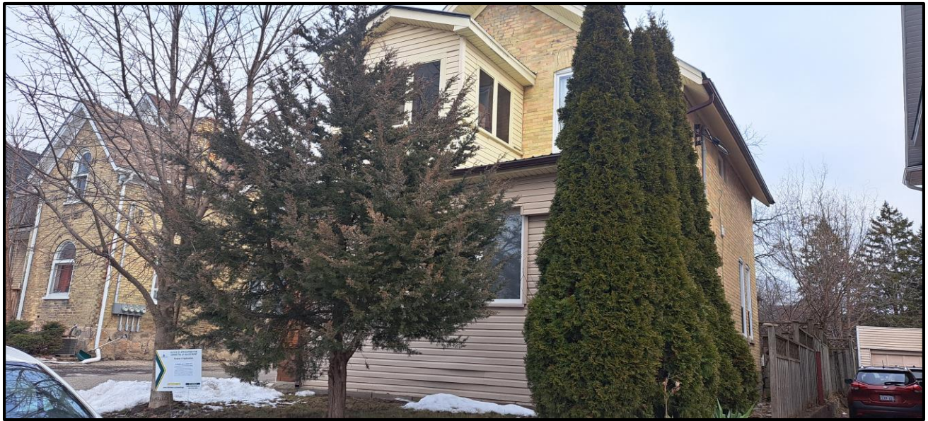
Figure 4: Front view of the existing single detached dwelling
