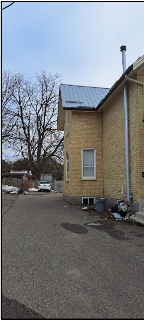
Figure 5: North side yard with the existing driveway
