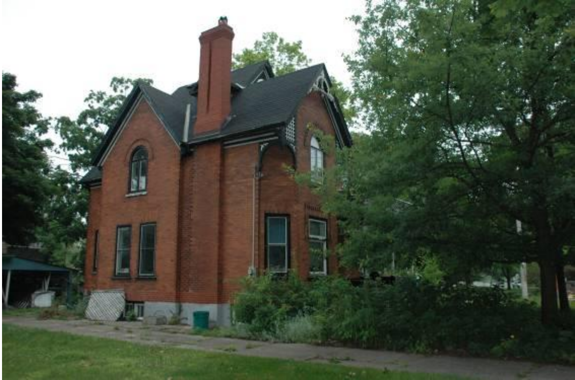
35 Courtland Avenue West – Side (East) Elevation
