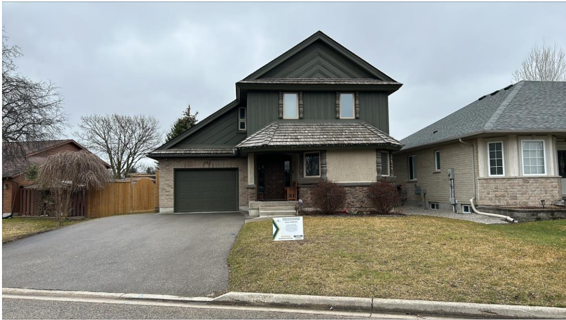
Figure 2: Front View of 167 Forfar Avenue
