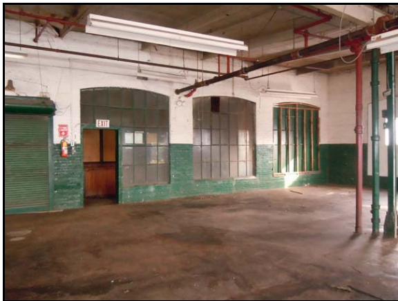
Figure 37 interior (east) 1913 wall
