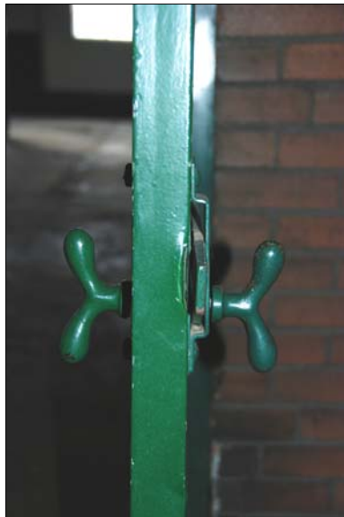
Fig. 33 door hardware at stairwell
