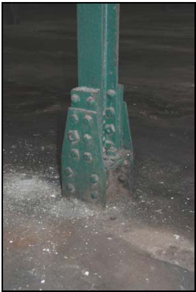
Fig. 32 riveted shear plate column
