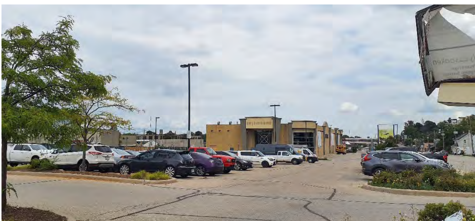
Figure 11: building located at 264 Victoria Street North (MHBC, 2023)
