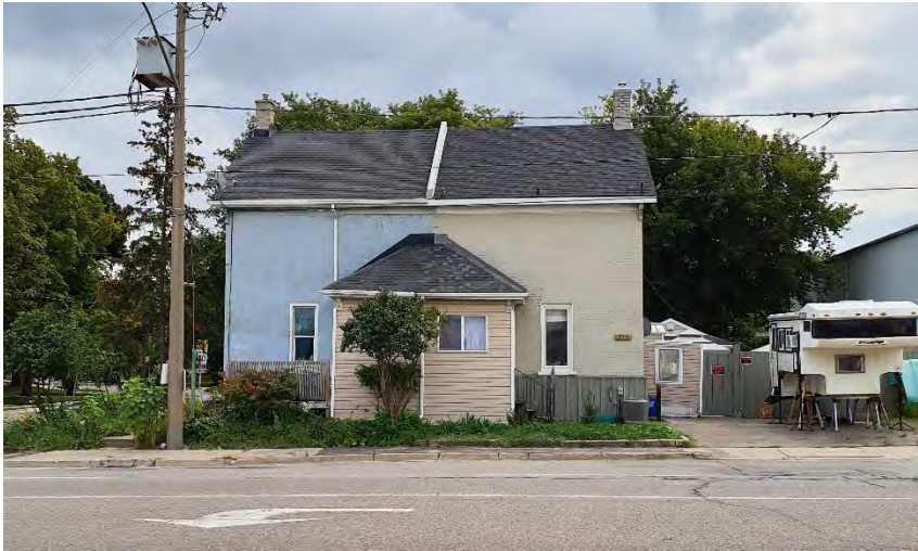
Figure 8: Side façade of 277 Victoria Street (in blue) (MHBC, 2023)
