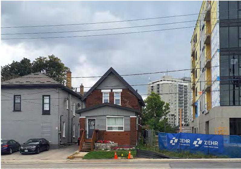
Figure 5: front façade of 231 Victoria Street (MHBC, 2023)
