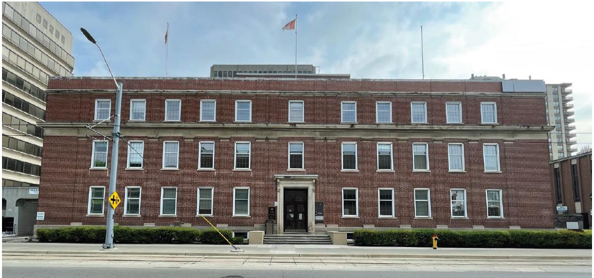
Figure 1: Front (South) Facade of Subject Property
