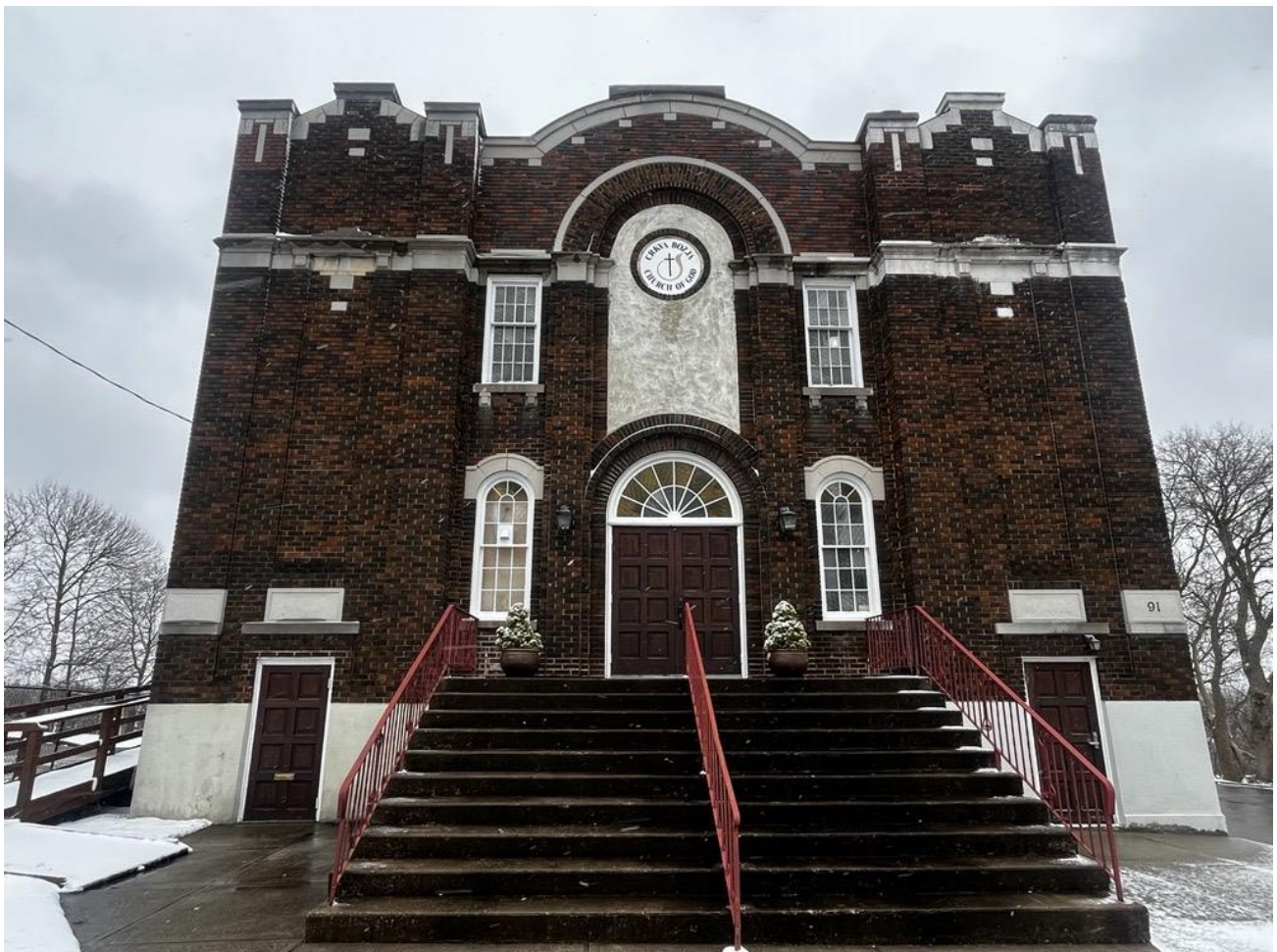
Figure 2: Front Façade of Subject Property
