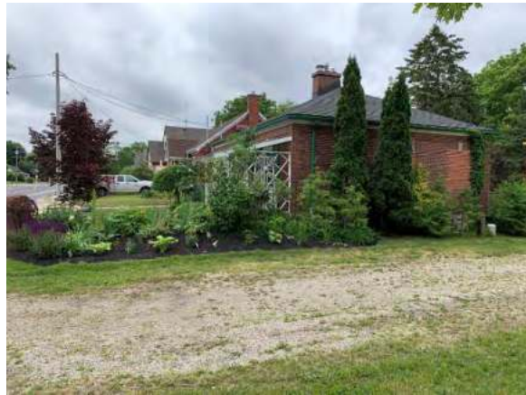
Photo 2: General view of gravel lane and buildings, facing east
