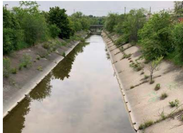
Photo 16: General view of Schneider Creek with concrete embankments, facing northwest
