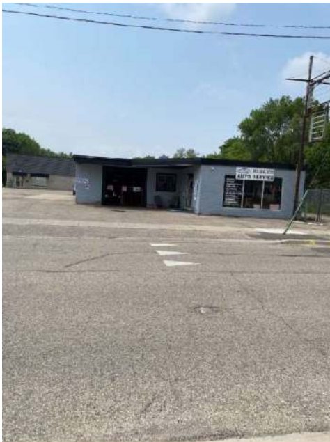
Photo 3 – View of auto service garage at 116 Kent Avenue, facing northwest.
