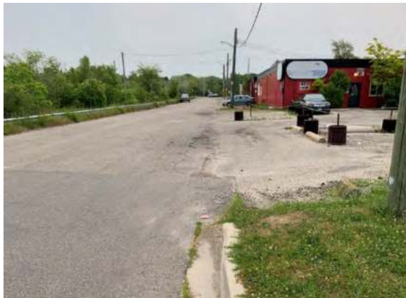
Photo 15: General view of street and existing buildings, facing southeast
