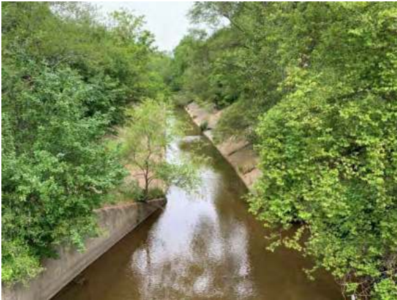
Photo 11: General view of Schneider Creek with concrete embankments, facing northwest
