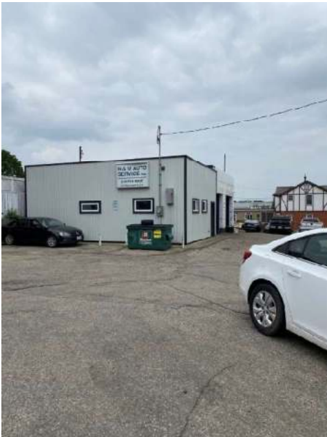
Photo 7 – Auto service garage at 440 Courtland Avenue East, facing north.
