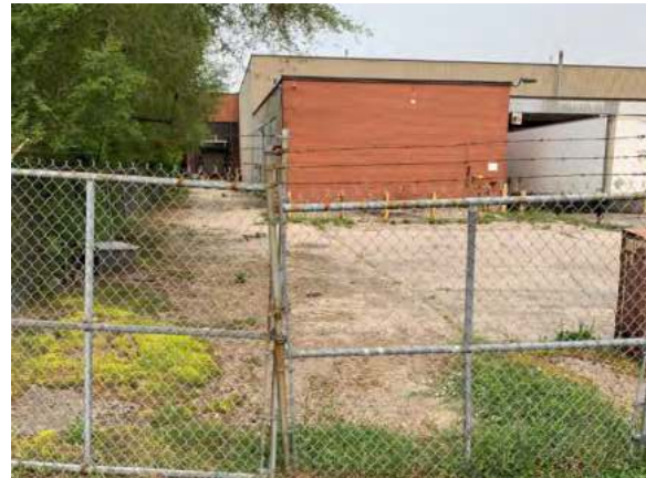
Photo 14: General view of existing buildings and parking lot, facing northwest
