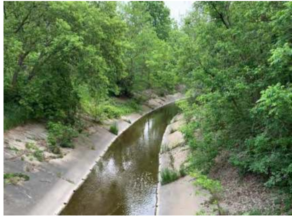
Photo 6: General view of Schneider Creek with concrete embankments, facing east
