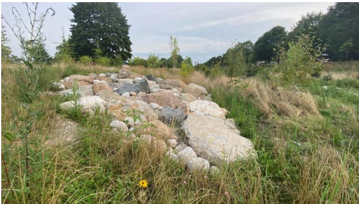
Photo 3.2: Boulder Step-Down Feature at Montgomery Creek
