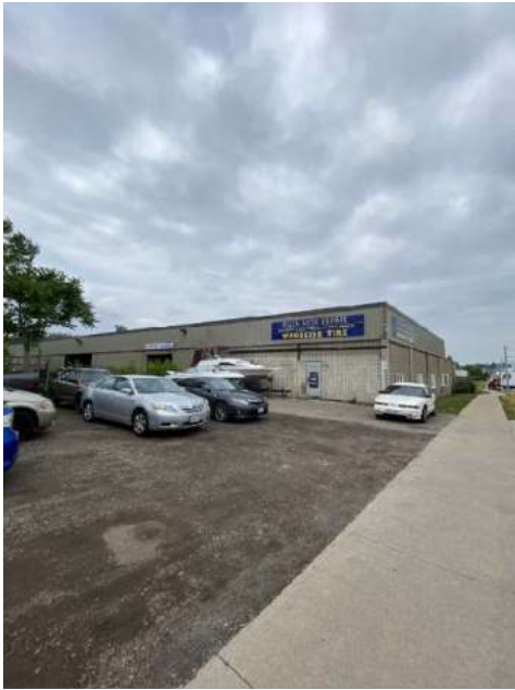
Photo 1 – View of 170 Borden Avenue South, facing north.
