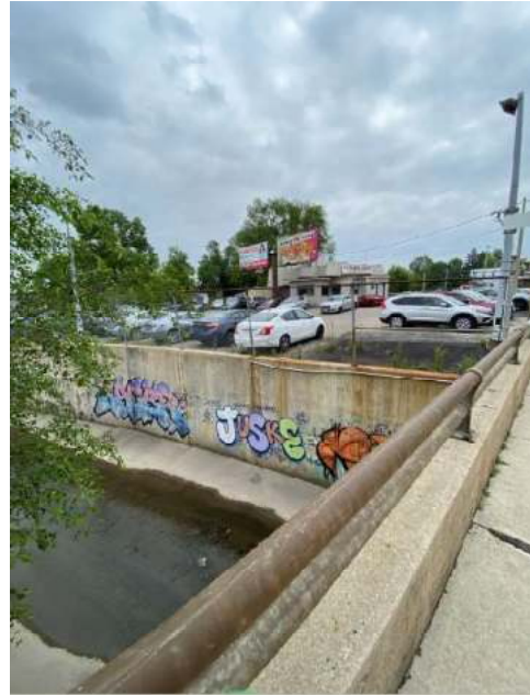
Photo 10 – View of Shoemaker Creek at Courtland Avenue East, facing northeast.
