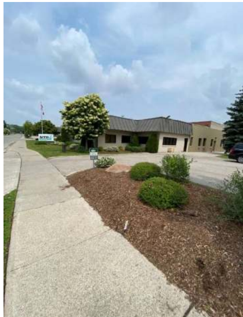
Photo 4 – View of 97 Kent Avenue, facing east.
