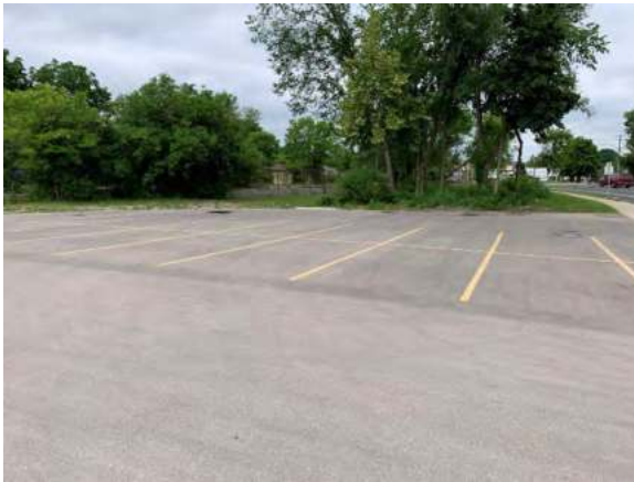
Photo 1: General view of paved parking lot, facing southwest
