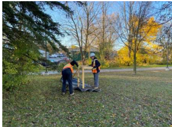
Photo 4: Test pit survey, facing north
