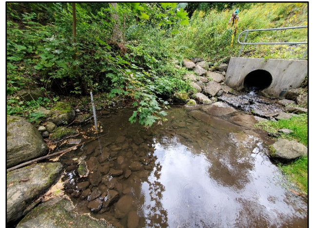
Photo 10. Hidden Valley Road Crossing, downstream view
