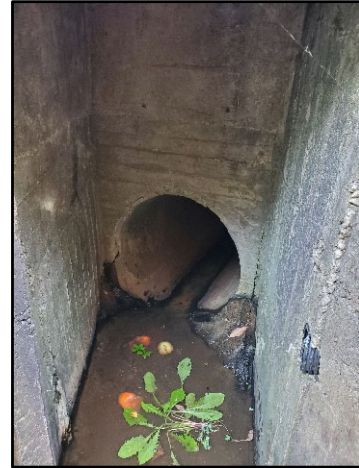
Photo 14. 735 Hidden Valley Road Driveway low flow culvert, view upstream
