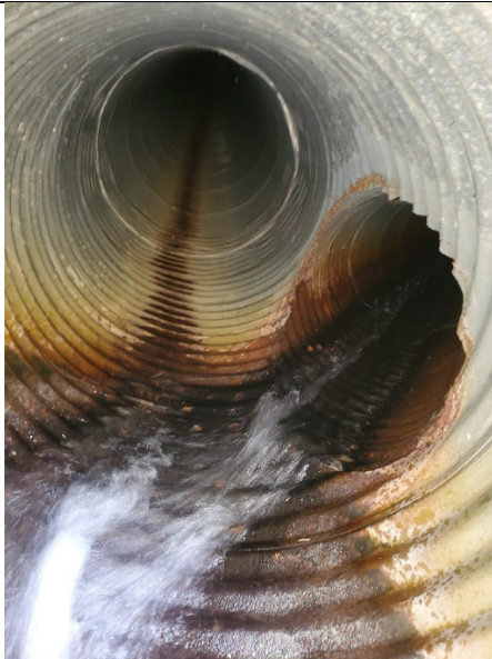
Photograph 3: View of pipe confluence under Hidden Valley Road.
