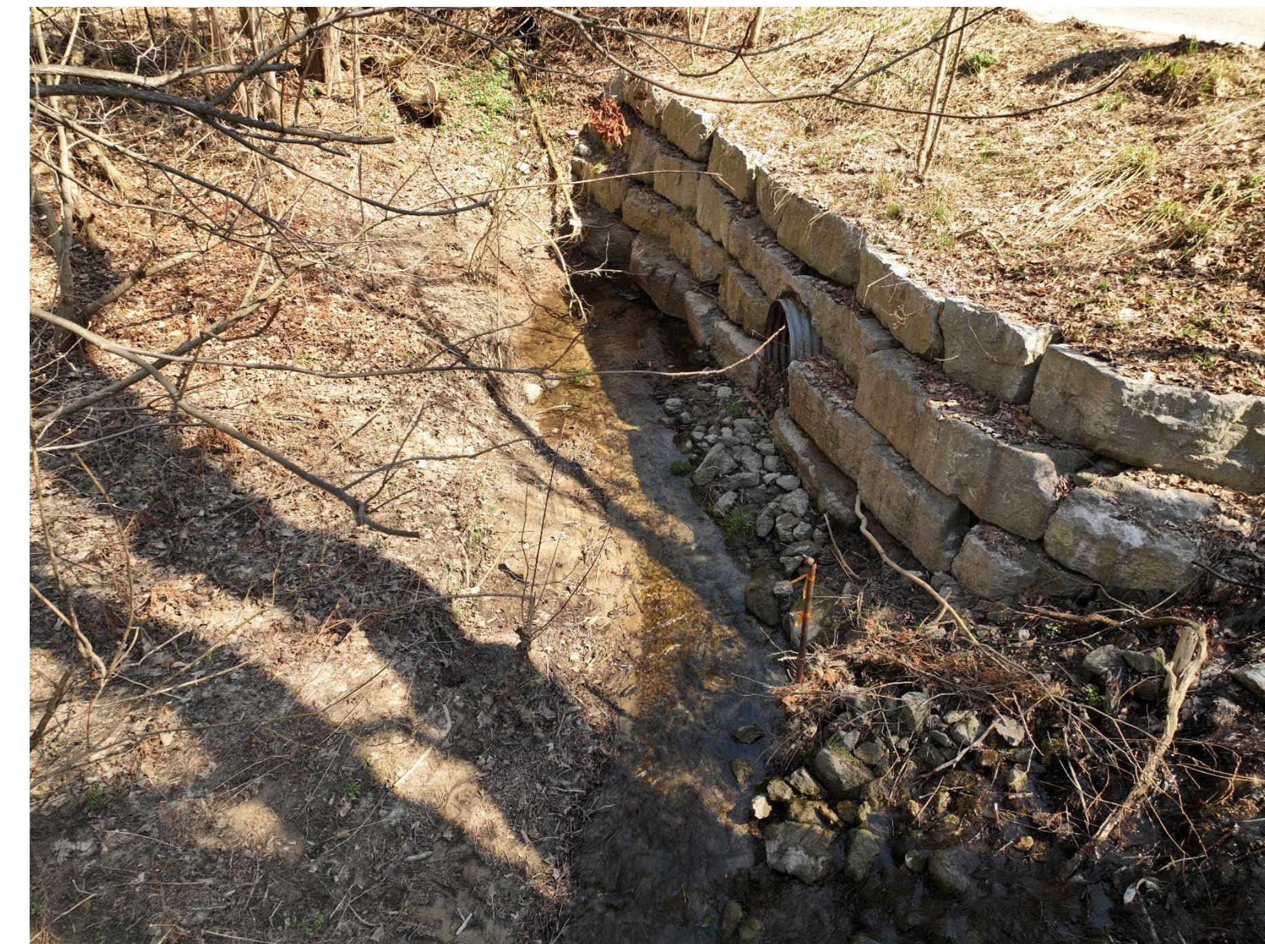
Headwall of Hidden Valley Road crossing; note almost complete submersion of northern culvert by sedimentation
