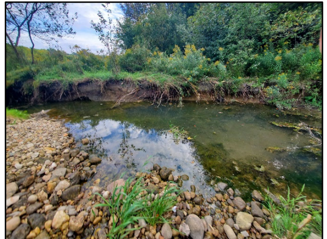
Photo 4. Hidden Valley West Creek naturalized banks with undercutting
