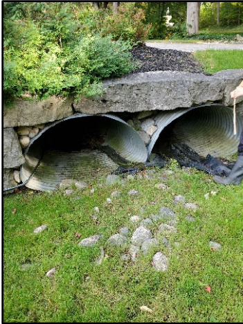
Photo 13. 735 Hidden Valley Road Driveway bypass culverts, view upstream
