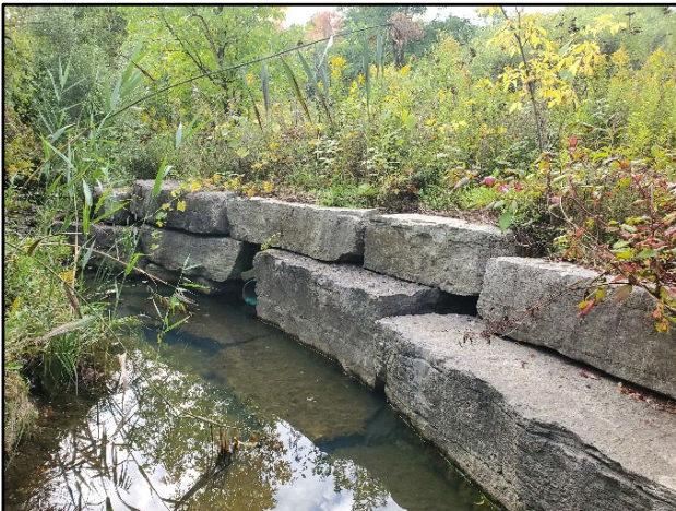
Photo 3. Hidden Valley West Creek armour stone bank
