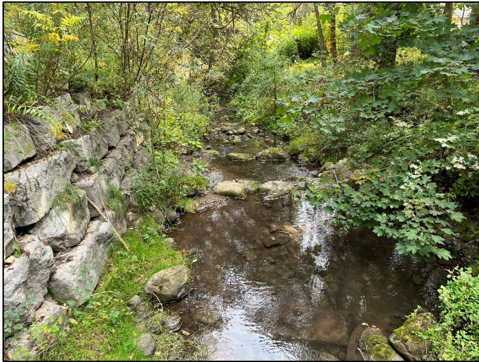
7. Hidden Valley Creek. Immediately downstream of the Hidden Valley Road culvert.
