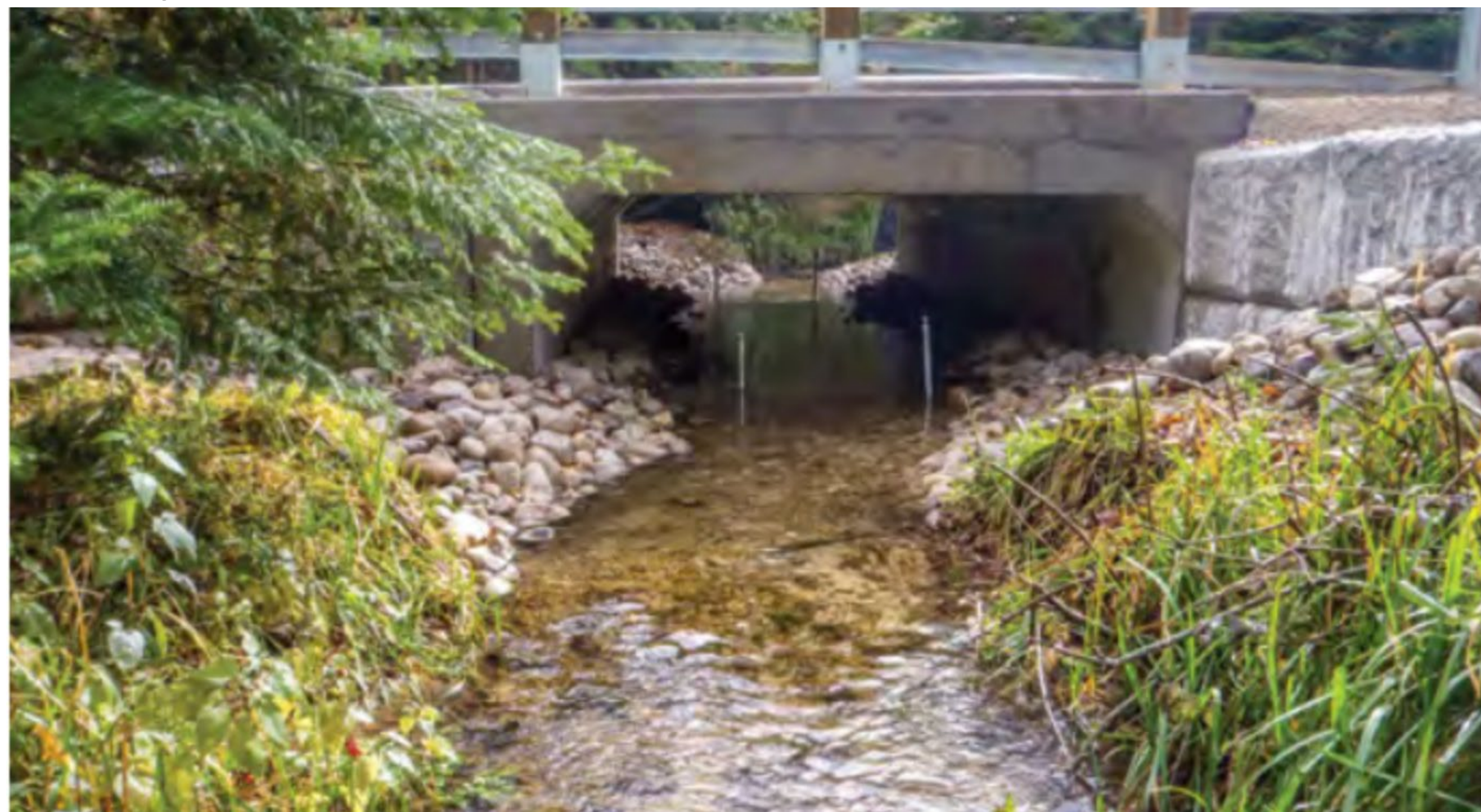
Example Box Culvert
