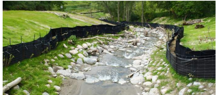
Example Watercourse Stabilization
