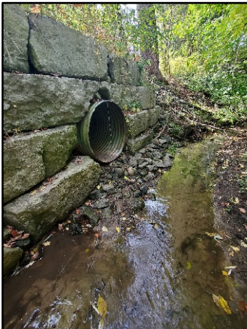
Photo 9. Hidden Valley Road Crossing, upstream view
