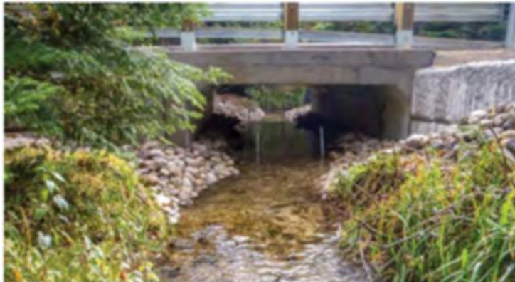
Example Box Culvert
