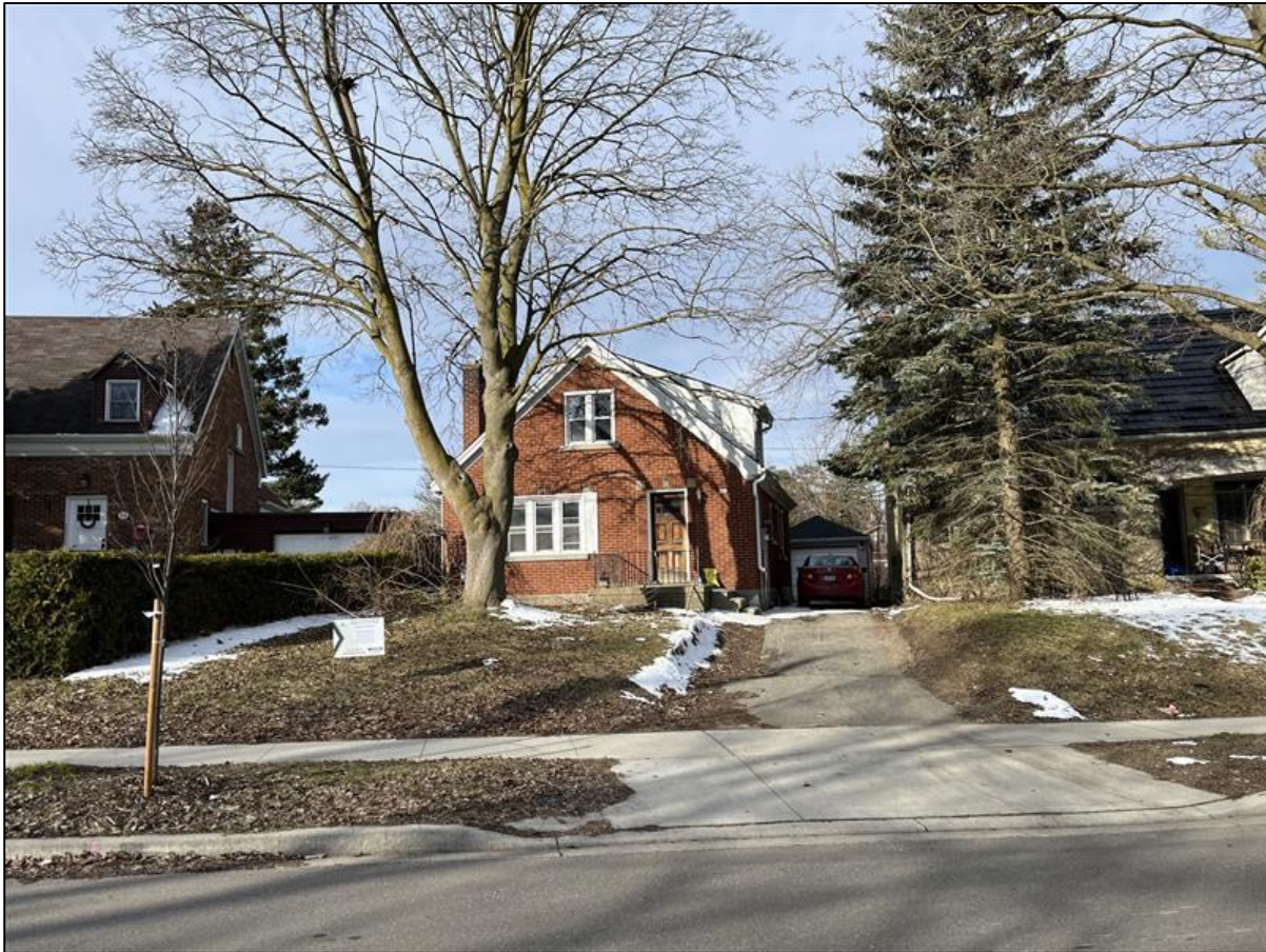
Figure 2: View of Existing Single Detached Dwelling (March 25, 2024).
