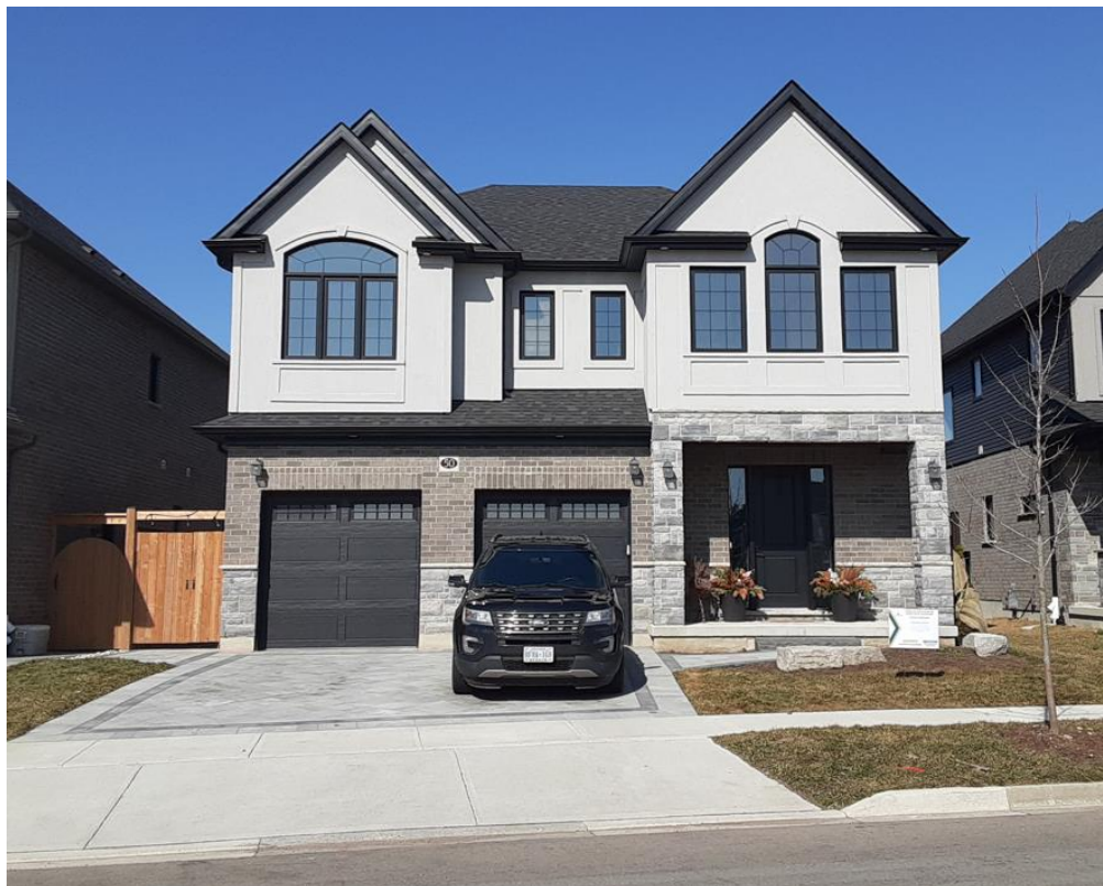
Figure 3 - View of property from street.
