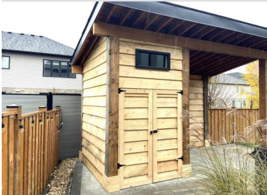
Figure 5 - View of accessory structure from the left side.
