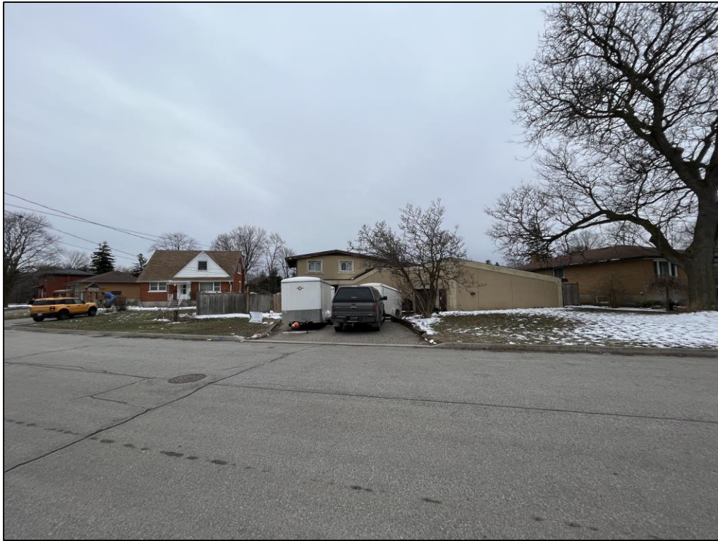
Figure 2: View of Existing Single Detached Dwelling (March 22, 2024).
