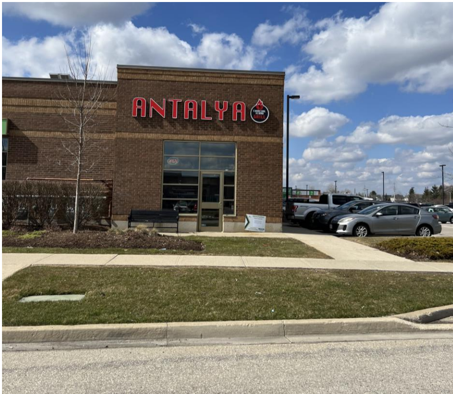
Figure 2 – Site visit photo of proposed patio location.
