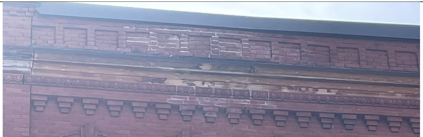
Third-storey details showing highly decorative brick cornice, brick frieze, and stone and brick architrave; and, ornamental brick moulding along with red brick corbelling – 83-85 King Street West
