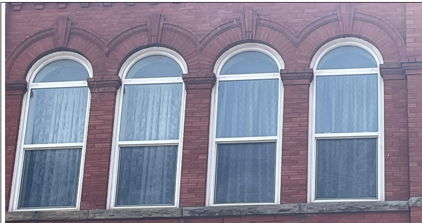
Third-storey details showing semi-circular window openings; semi-circular transom design; and, 1/1 hung window design with brick voussoirs and continuous stone sills
