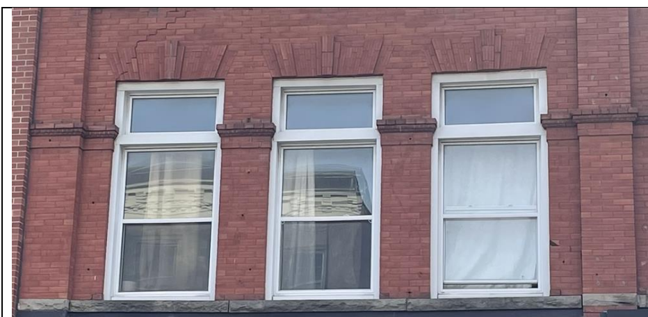
Second-storey details showing flat head window openings; rectangular transom design; and, 1/1 hung window design with brick voussoirs and continuous stone sills
