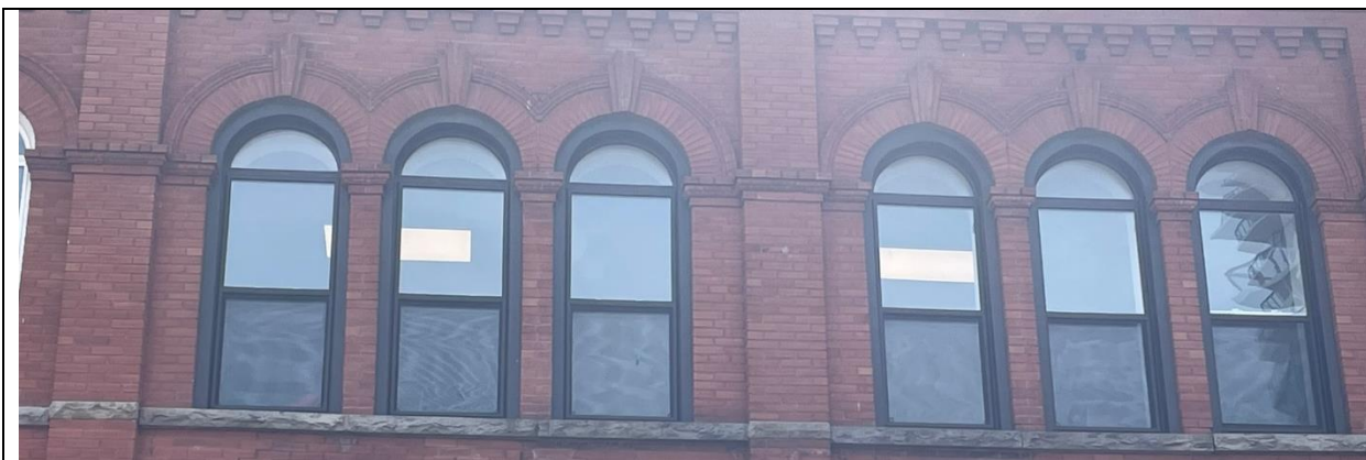
Detailing of third-storey semi-circular window openings; semi-circular transom design; 1/1 hung window design featuring decorative brick hood moulds with keystones and continuous stone sills
