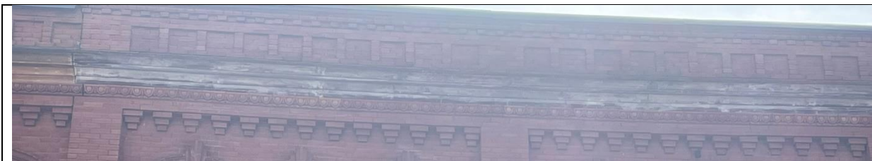
Detailing of brick frieze, stone and brick architrave and ornamental brick moulding along with red brick corbelling
