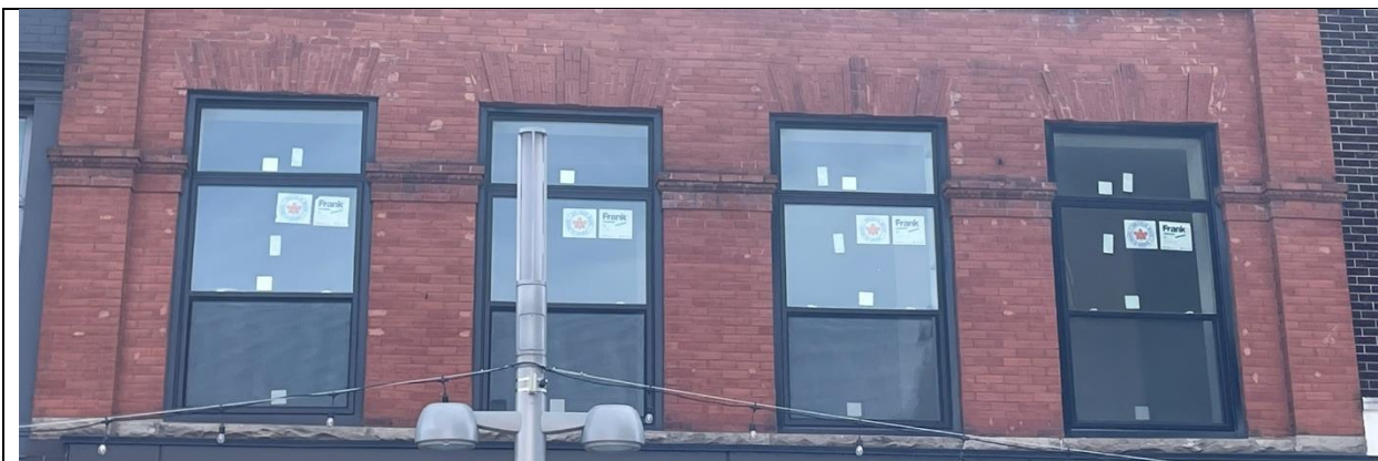
Detailing of second-storey showing flat head window openings; rectangular transoms; 1/1 windows; and, brick voussours and continuous stone sills
