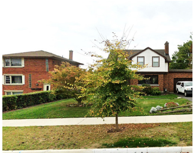
Figure 3.2 - Residential dwellings along Fairmount Road (North)
