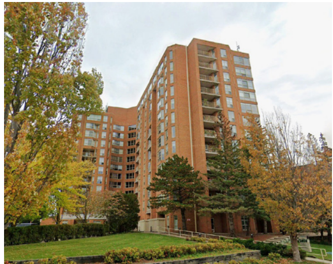
Figure 3.7 - High-rise apartment dwellings at 1414 King Street E
