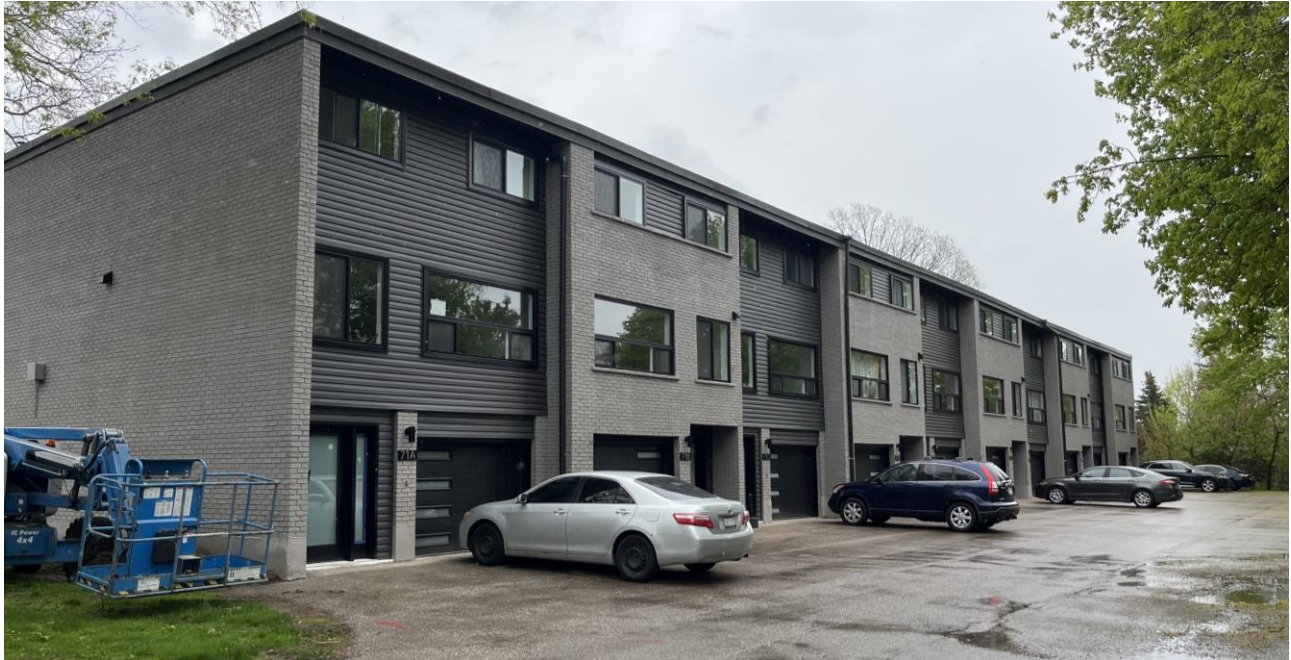
Figure 3 – Existing rear building – 71 Blucher Street
