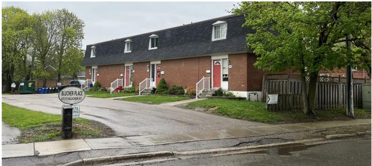
Figure 2 – Existing front building – 67 Blucher Street
