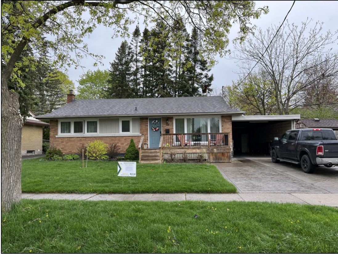
Figure 2: View of Existing Single Detached Dwelling (May 3, 2024)
