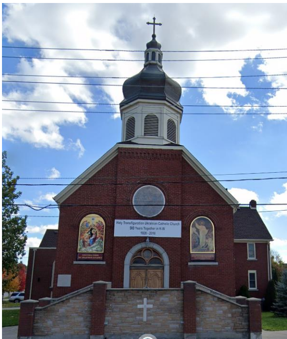
Figure 2: Front Elevation (West Façade) of the Subject Property – 131 Victoria Street South (Ukrainian Catholic Church of the Transfiguration)
