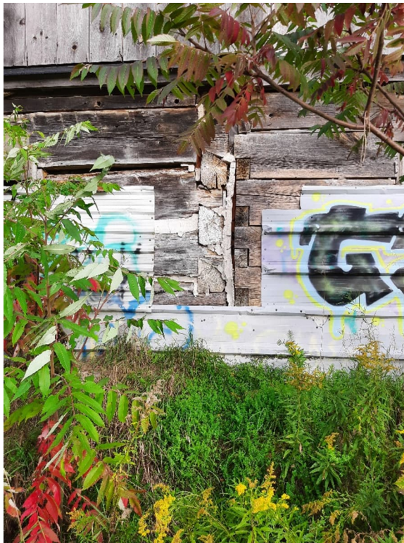
Photograph No. 23 – Wall Joinery Indicates Staged Construction
