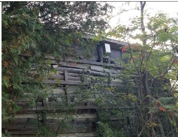
Figure 23: Original log house (west elevation) showing original logs and mortar (MHBC).
