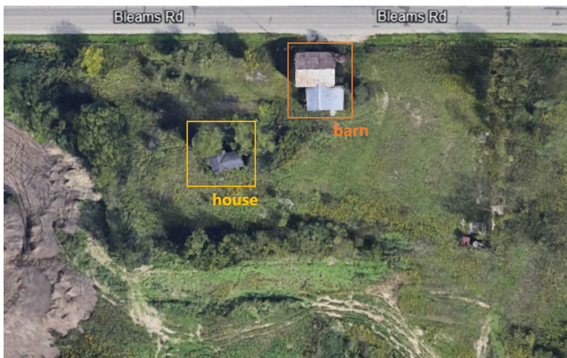
Figure 11: current condition of subject property (Google, 2023)
