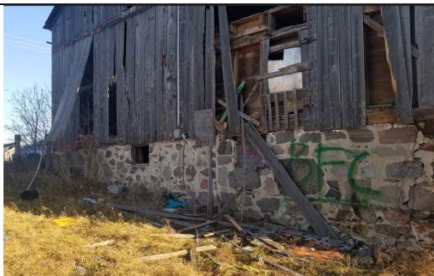
Figure 16: Fieldstone foundation along the west elevation (MHBC, 2023)
