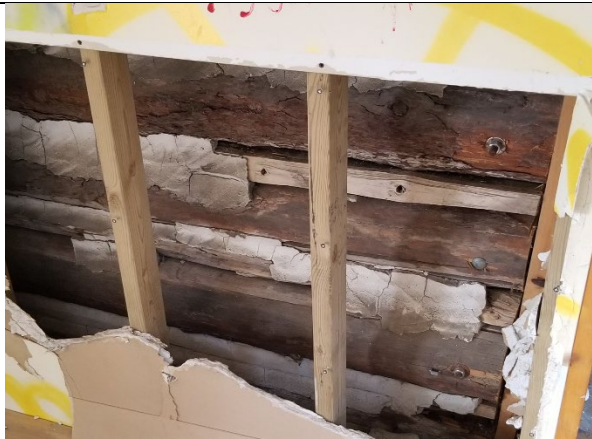
Figure 26: Interior photograph of the original logs and mortar (MHBC).
