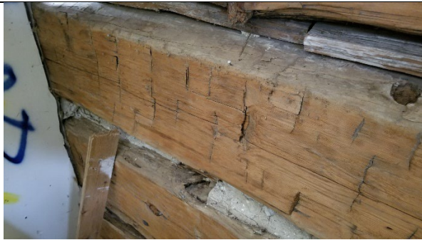
Figure 25: Interior photograph of the original hand-hewn timber (MHBC).
