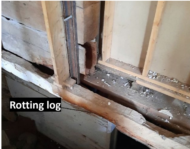
Missing post and disconnected support beam
