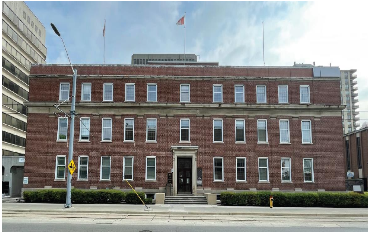
Figure 2: Front (South) Facade of Subject Property
