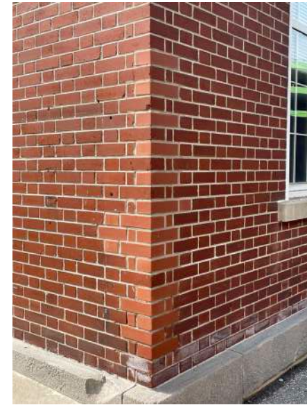
Figure 11. Detail of the Queen Street Facade (left) and right side of the rear facade (right) showing locations where efflorescence and mortar deterioration has occurred due to water damage. (Source: mCs, July 2021)
