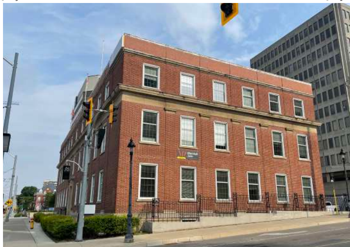
Figure 12. Perspective View of the subject property from Duke St W and Queen St intersection showing the heritage attributes of the building: 11 bays along Duke and 6 bays along Queen, the concrete band between the 2nd and 3rd floors, the parapet at the roofline with red brick on all facades. (Source: mCs, July 2021)
