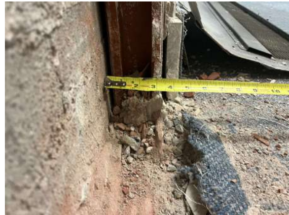
Fig 10: Add'l removals of interior finishes at slab level
