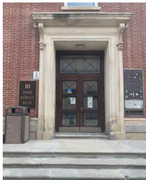
Figure 10. Detail of the front facade fronting Duke Street West showing the main entrance door with door surround paneled glass and transom and entablature above. (Source: mCs, July 2021)
