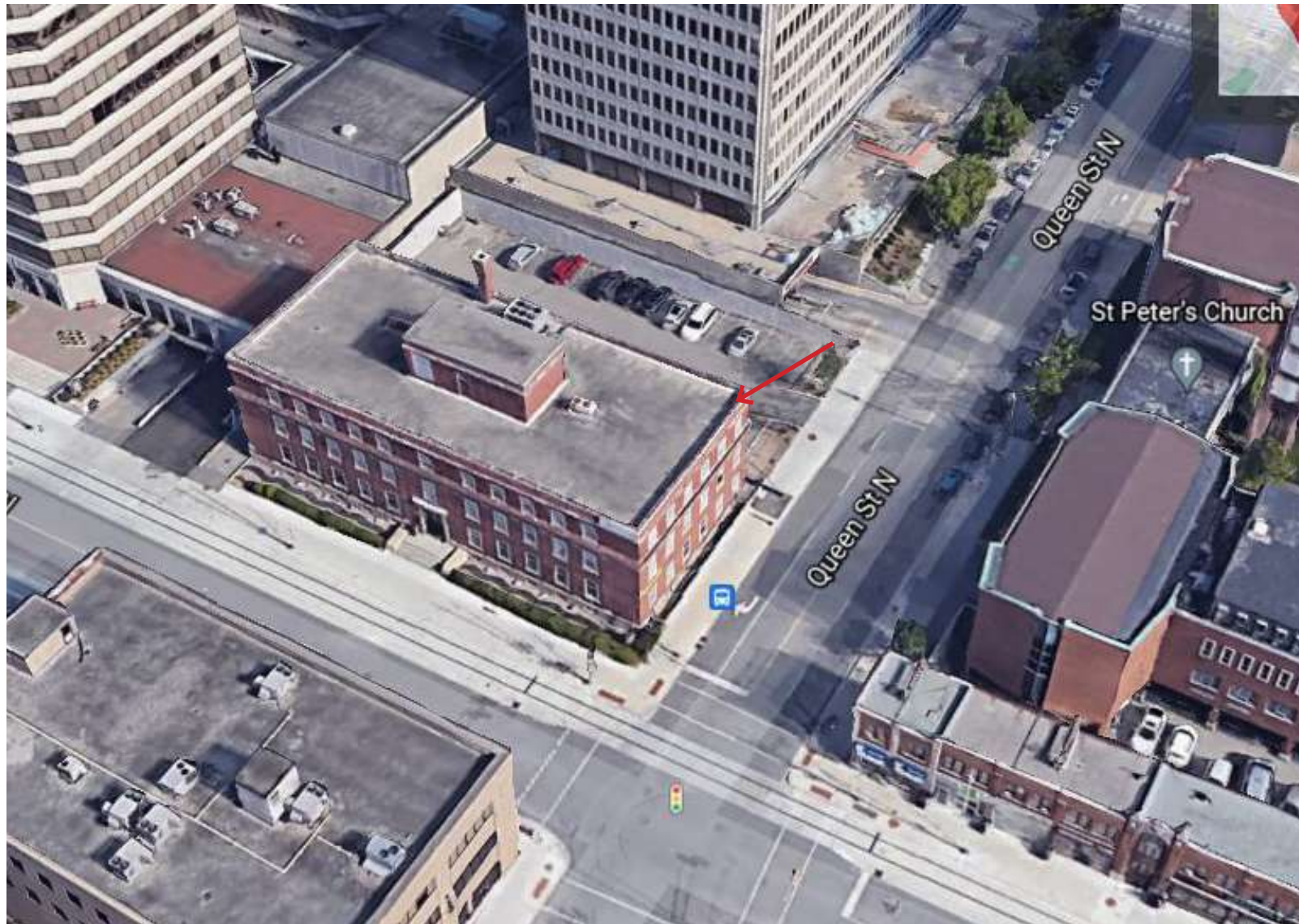
Figure 1. Aerial View Image showing the location of 10 Duke Street W at the corner of Queen and Duke in Downtown Kitchener, ON. (Source: Google Earth). Annotated by mCs to show the subject site.
